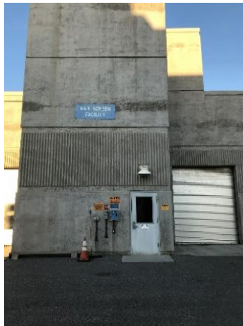
Photo of Plant No. 2 Screening Area
