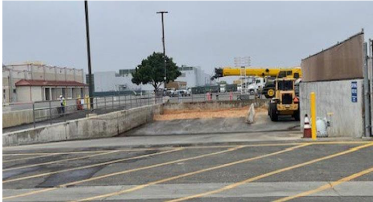
Photo of Plant No. 1 Drying Beds Area
