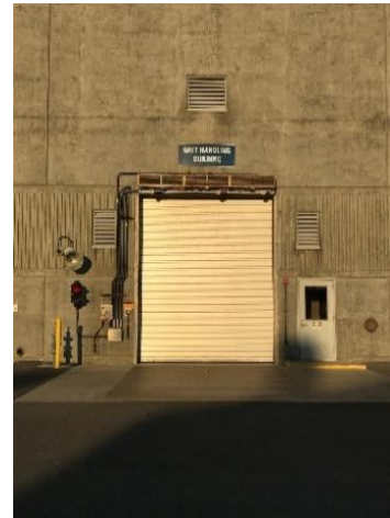
Photo of Plant No. 2 Grit Area
