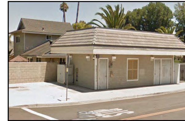
College Pump Station
