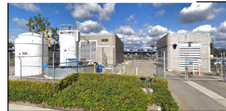
Main Street Pump Station
