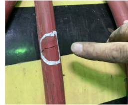
Cracked generator cable leads
