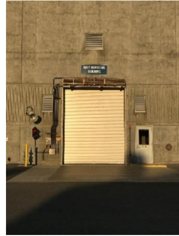
Photo of Plant No. 2 Grit Area
