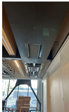
Chilled Beams
