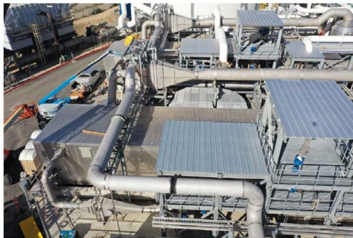
Figure 7: Dryer Installation at RBF
