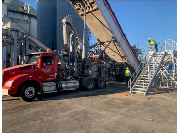
Figure 6: Truck Unloading at RBF
