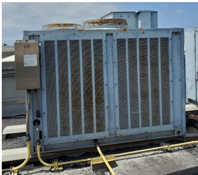
Figure 2: The Effluent Pump Station Annex (EPSA) electrical building HVAC units are experiencing signs of wear and failure.
