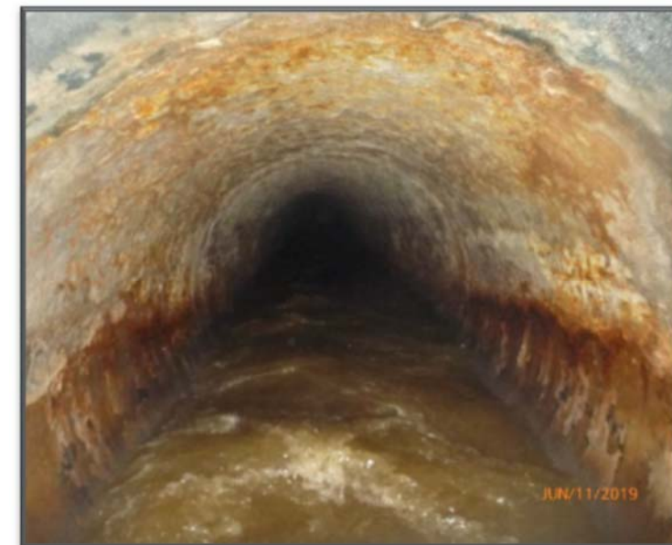
Santa Ana Trunk Sewer
