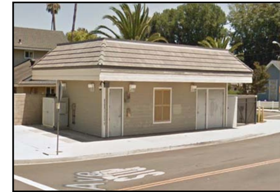
College Pump Station
