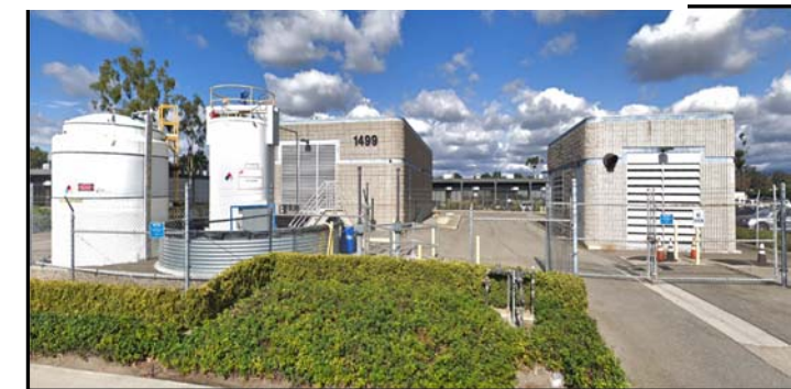
Main Street Pump Station
