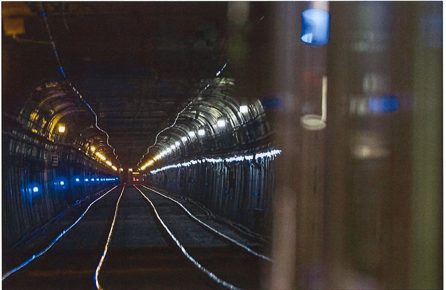
The Twin Peaks Tunnel
