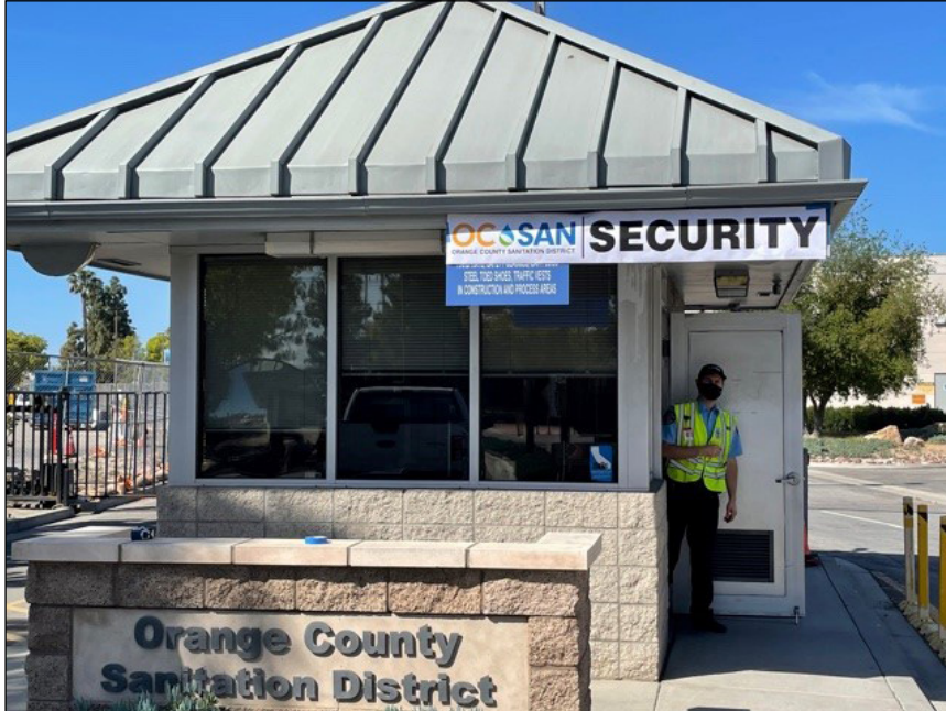
Plant No. 1 Security Booth Signage
