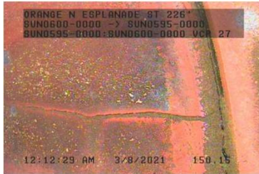
Cracked VCP pipe
