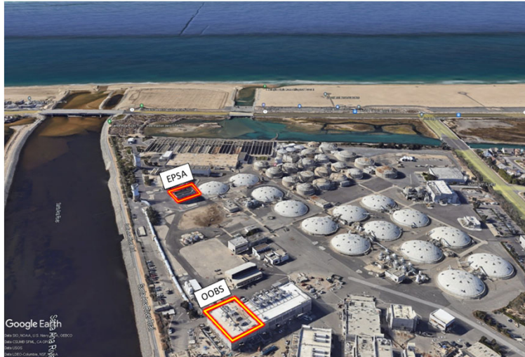
Plant No. 2 Aerial View
