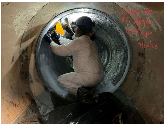
Full structural rehabilitation – Carbon fiber and fiberglass reinforced plastic with protective coating
