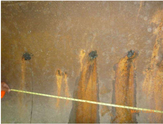
Holes discovered in existing 54-inch steel pipe (3/4-inch pipe wall thickness)
