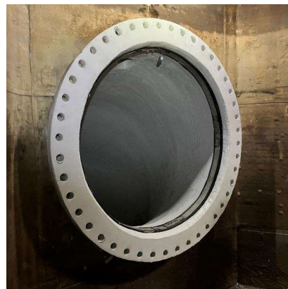
Full structural rehabilitation – Carbon fiber and fiberglass reinforced plastic with protective coating
