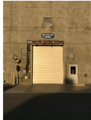
Photo of Plant No. 2 Grit Area
