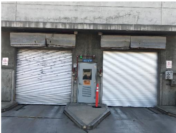
Photo of Plant No. 1 Grit and Screening Area
