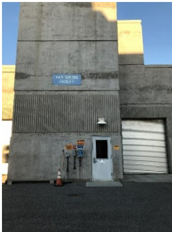
Photo of Plant No. 2 Screening Area
