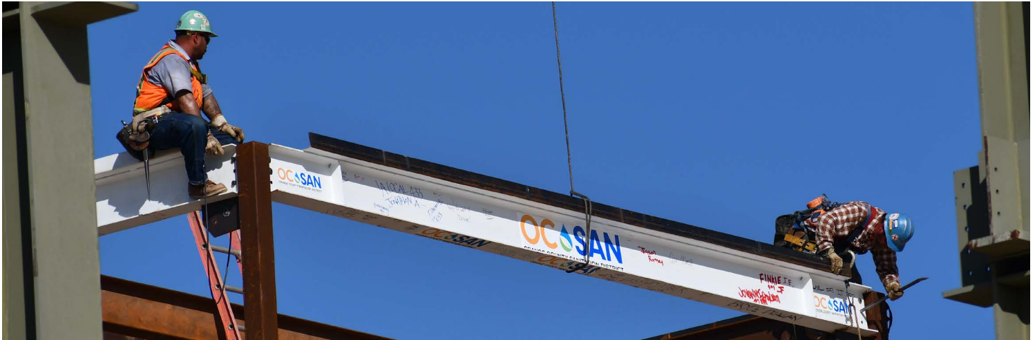
The last large structural steel beam is being installed.
