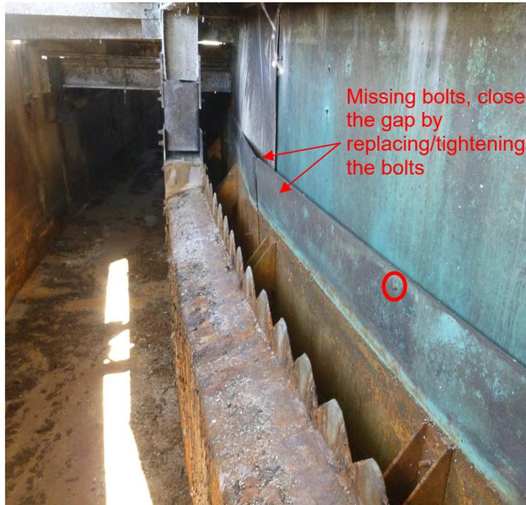
**Figure 13: Baffle Wall connection and missing bolts**
