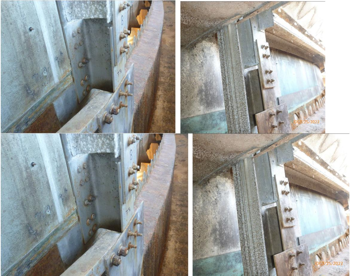
**Figure 8: Dome post typical configuration in Clarifier G**
