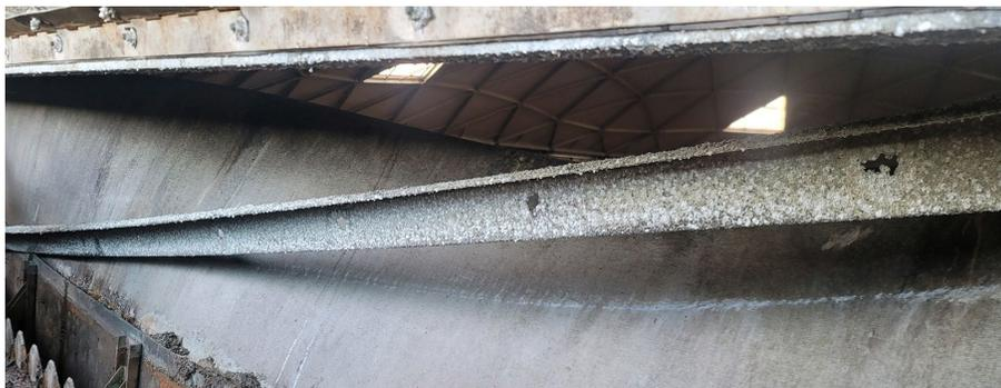
**Figure 4: Collapsed baffle wall and aluminum angle**
