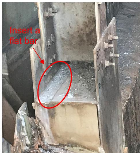
**Figure 6: Exposed steel plate (different basin)**
