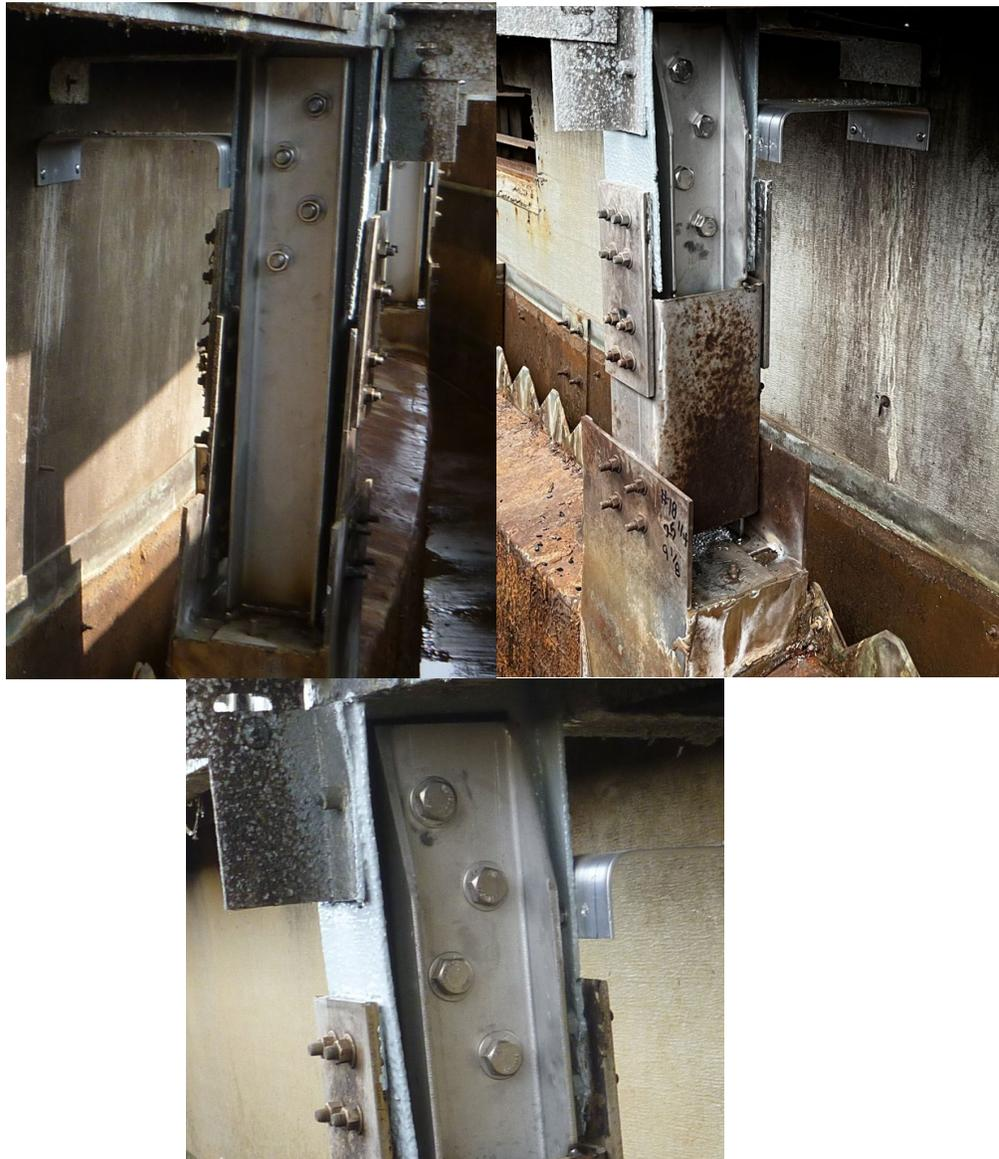
**Figure 7: Reinforced dome post (different basin) (typical)**
