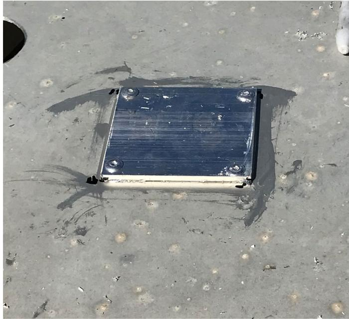
**Figure 20: Aluminum patch installed on top of a hole (different basin)**
