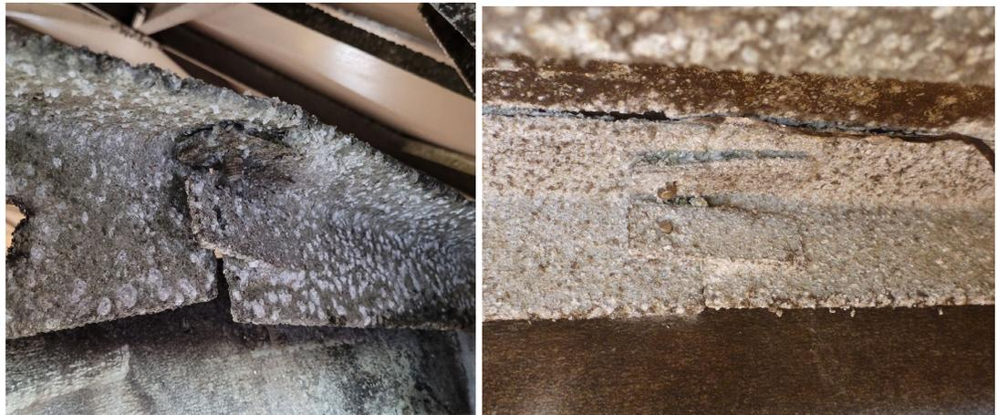
**Figure 14: Connector between two aluminum angles**
