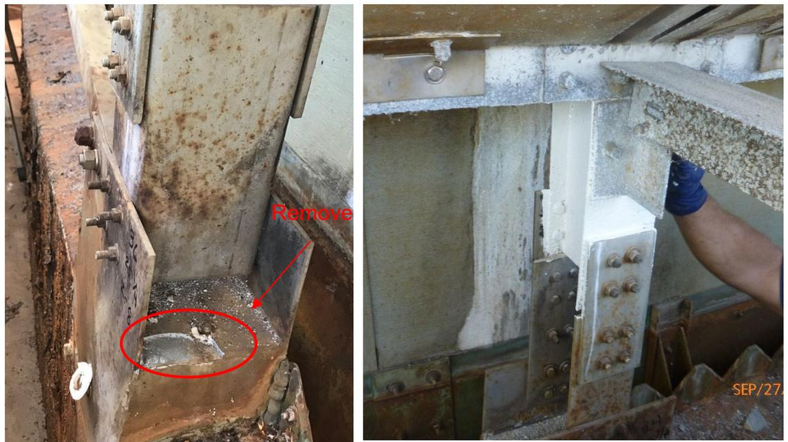
**Figure 5: Partially removed mortar liner above a steel plate (different basin)**
