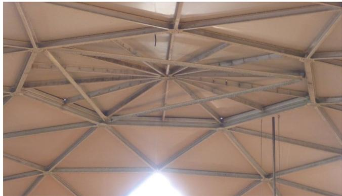
**Figure 15: Aluminum stiffeners below the removable dome hatch**
