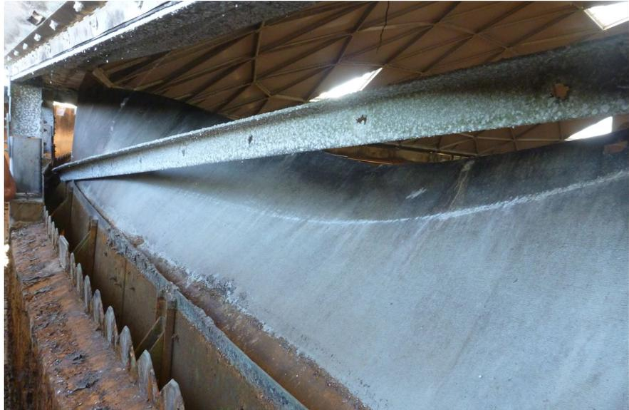
**Figure 12: Collapsed baffle wall in basin G**
