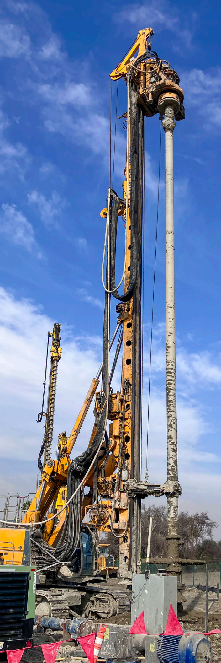
Cement-soil mixing drill rig used on the project.
