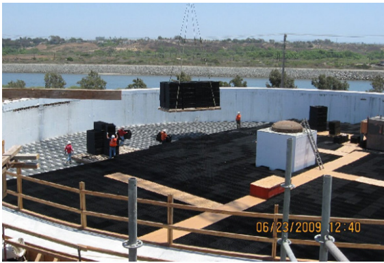
Construction of trickling filters.
