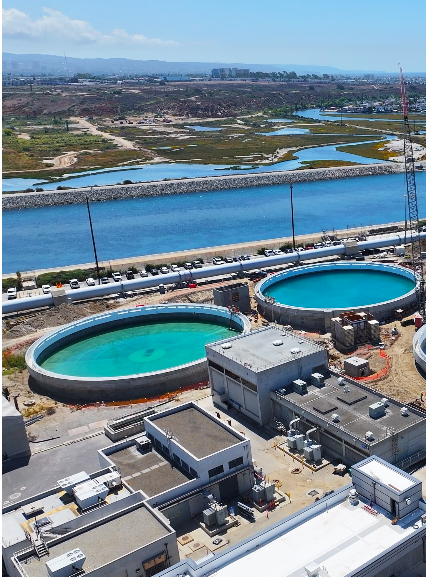
View overlooking the construction of four new primary clarifiers with the Santa Ana River and Newport Beach coast in the background.
