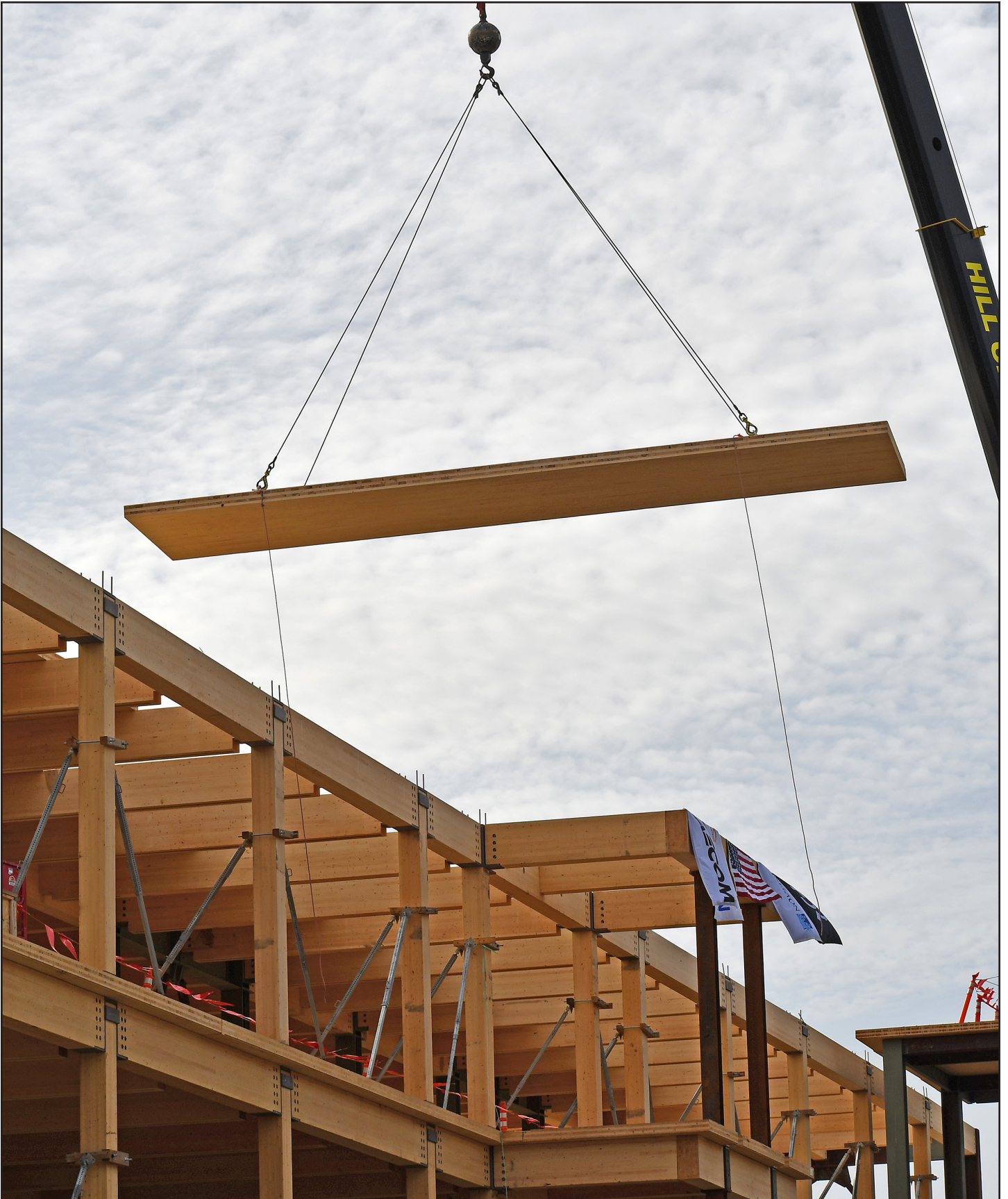
Final Mass Timber floor installation at future Headquarters Complex.
