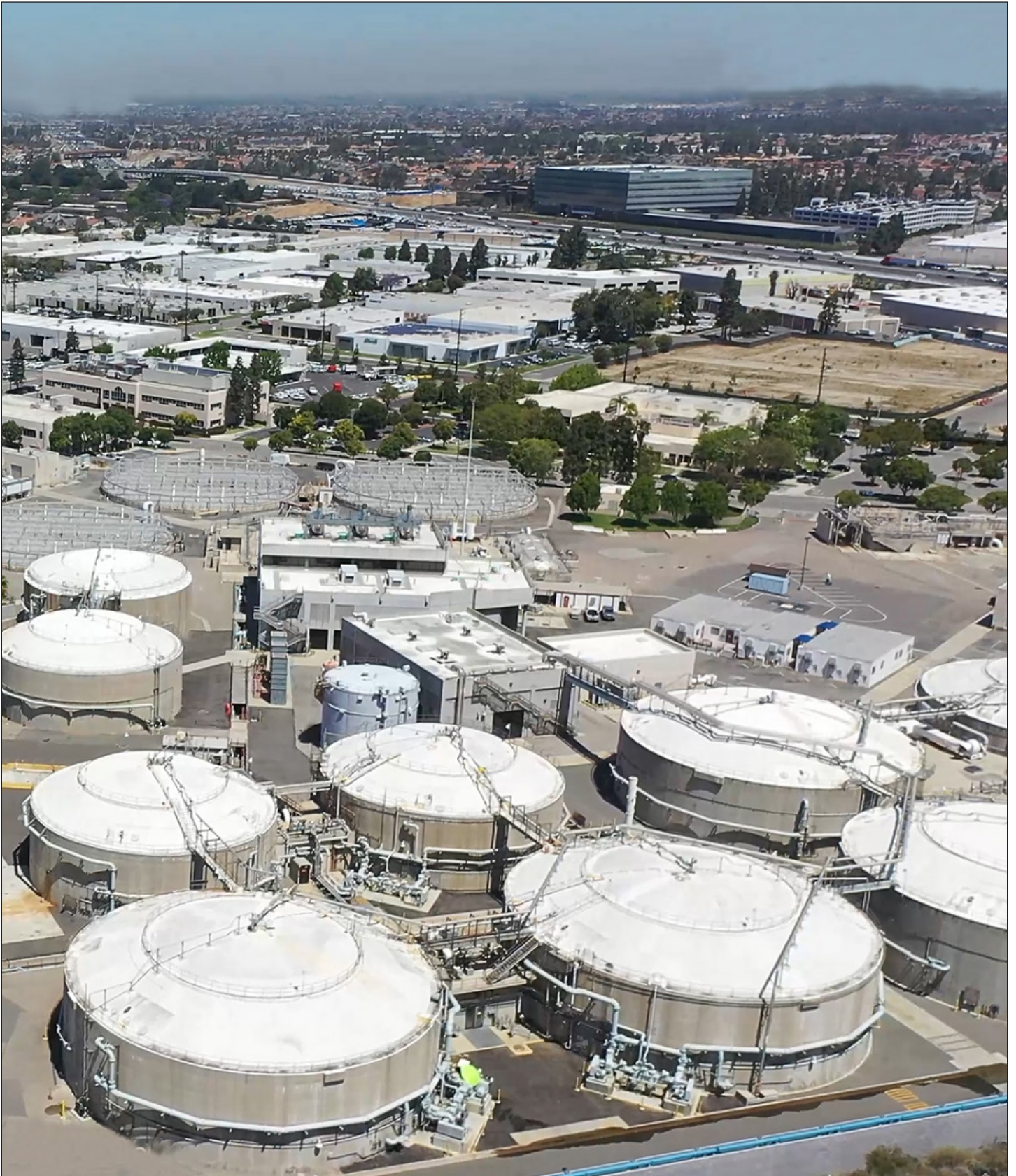
Reclamation Plant No. 1 in Fountain Valley.
