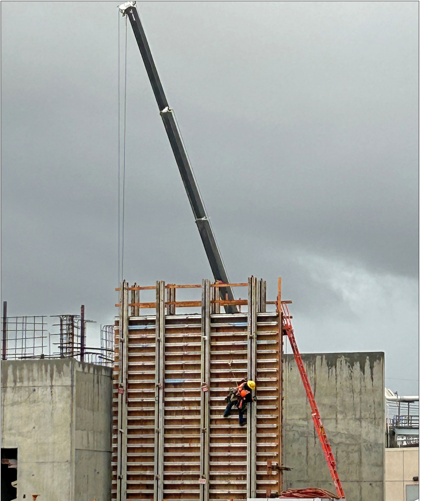
Headworks construction at Plant No. 1 in Fountain Valley.
