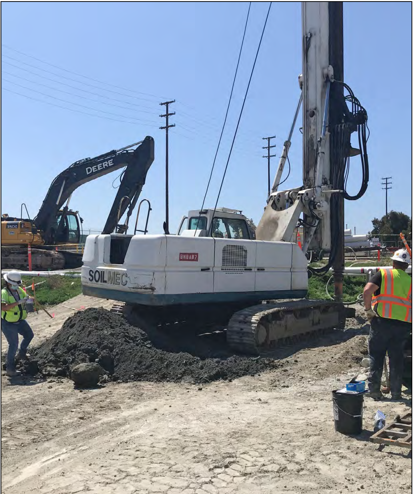
Redrilling well at Plant No.2 in Huntington Beach
