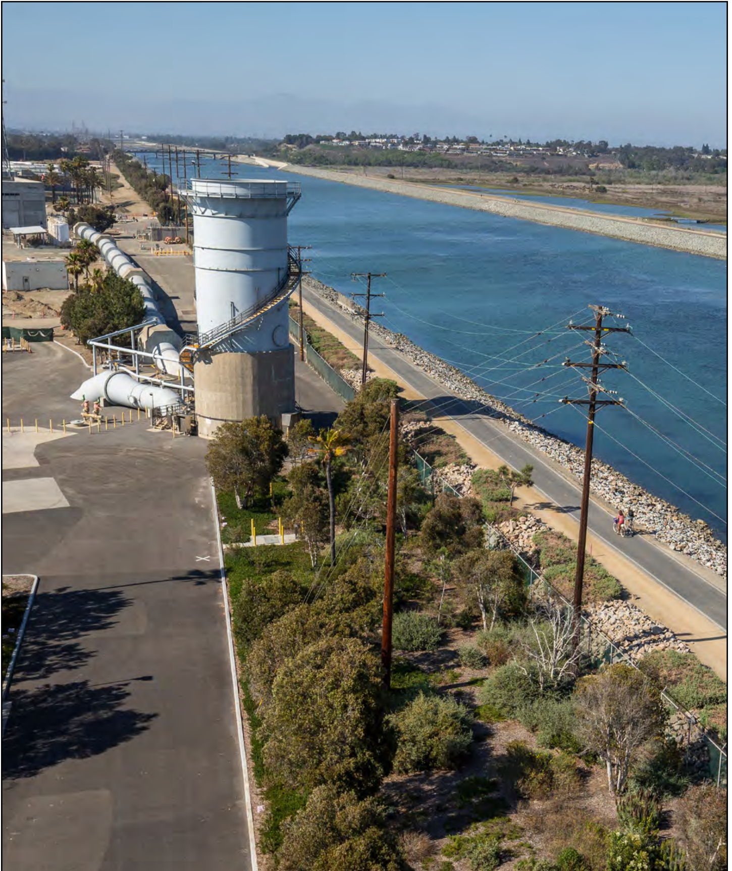
Surge Tower at Plant No. 2 in Huntington Beach
