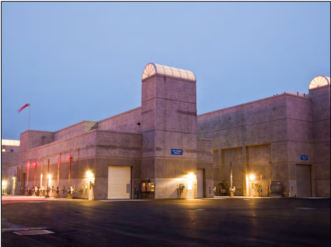
Bar Screen Facility and Influent Pump Station at Plant No. 2 in Huntington Beach
