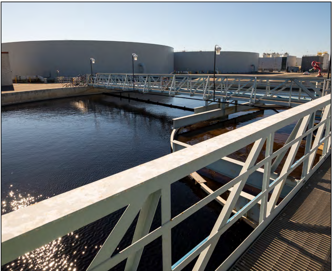
Trickling Filter and GWRS Tanks at Plant No. 1 in Fountain Valley
