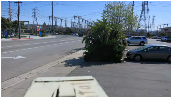
Noise Measurement Site L1 - looking east
