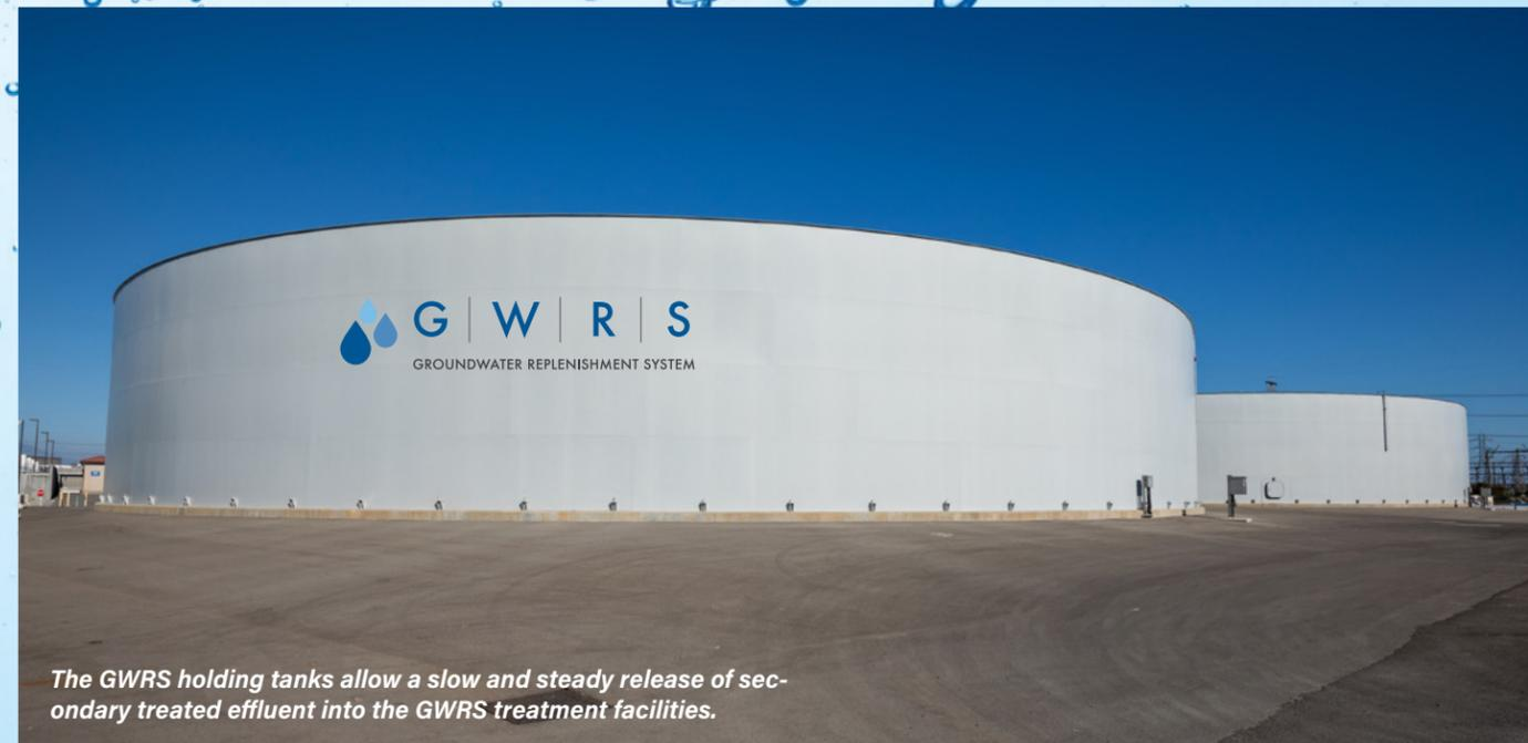
*The GWRS holding tanks allow a slow and steady release of secondary treated effluent into the GWRS treatment facilities.*
