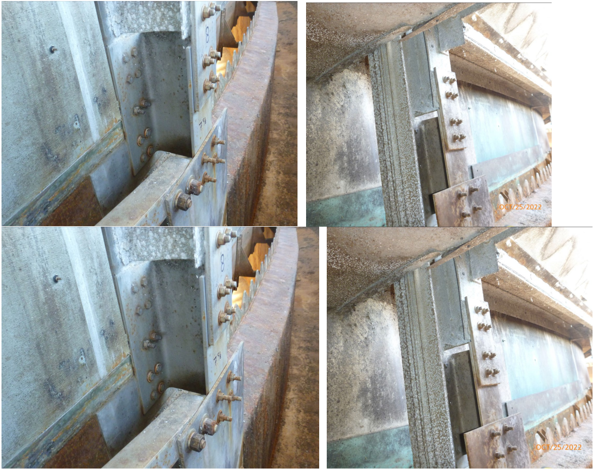
Figure 8: Dome post typical configuration in Clarifier G
