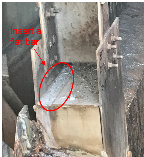
Figure 6: Exposed steel plate (different basin)
