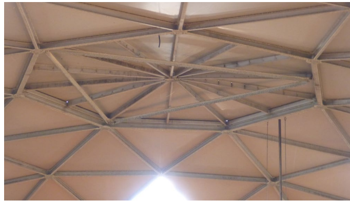
Figure 15: Aluminum stiffeners below the removable dome hatch
