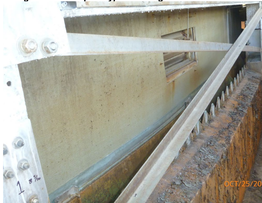
Figure 9: Dome post typical configuration in Clarifier G
