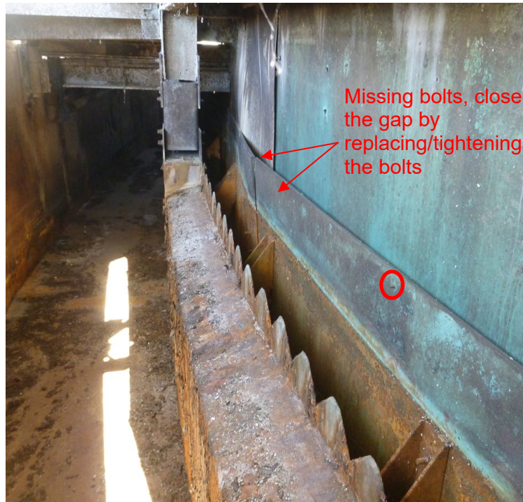
Figure 13: Baffle Wall connection and missing bolts
