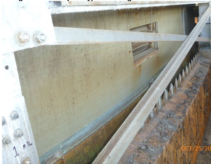
Figure 9: Dome post typical configuration in Clarifier G
