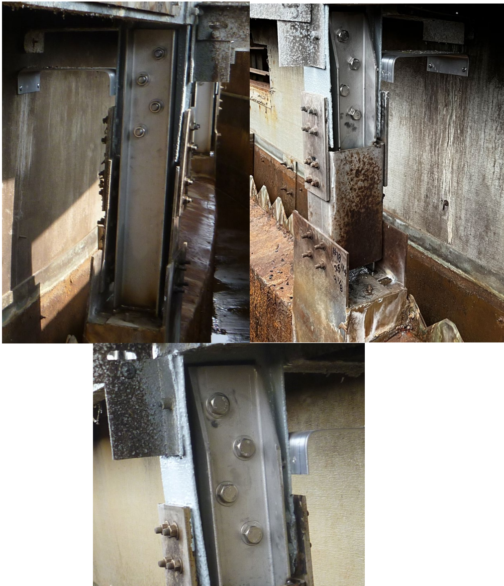
Figure 7: Reinforced dome post (different basin) (typical)
