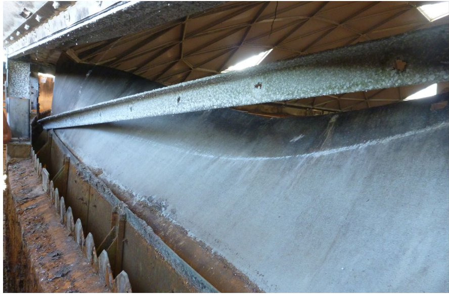
Figure 12: Collapsed baffle wall in basin G
