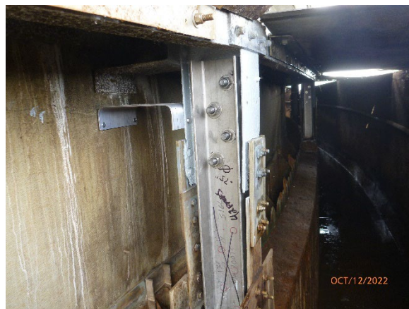
Figure 10: Aluminum angle and “Z” clip providing support to the baffle wall (Typical)
