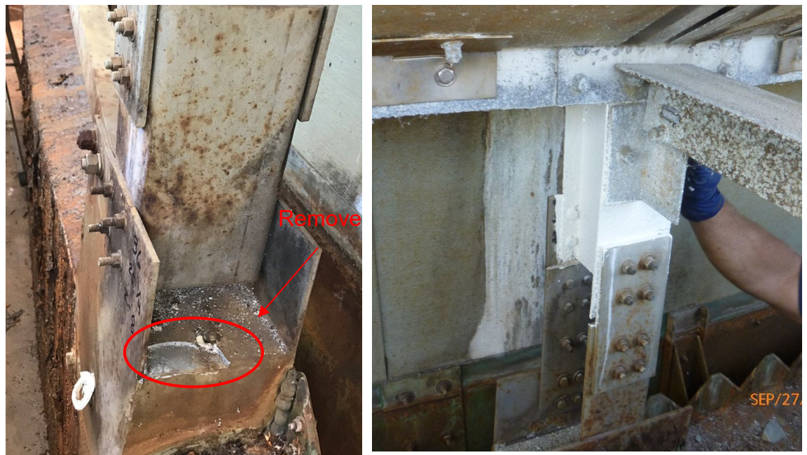
Figure 5: Partially removed mortar liner above a steel plate (different basin)
