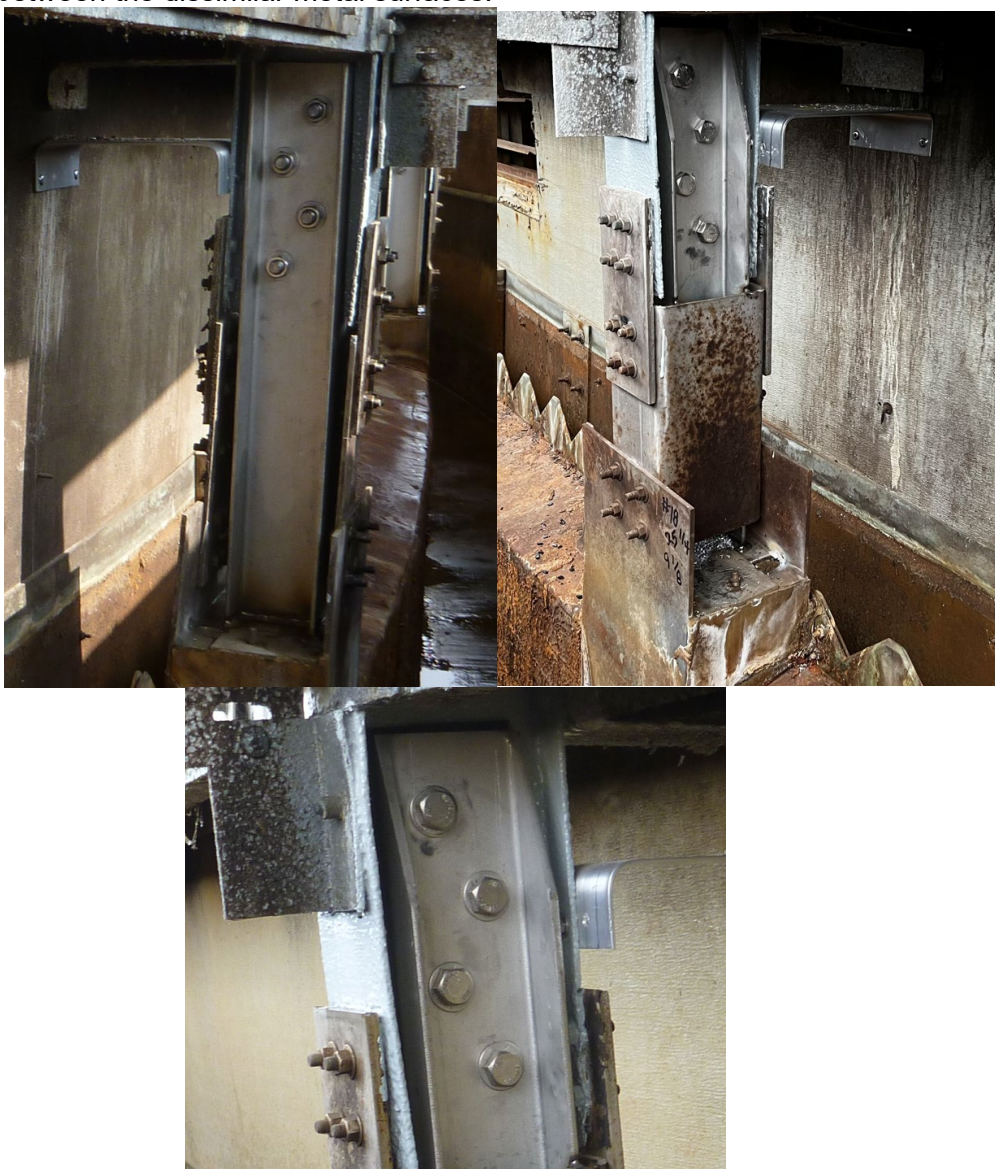
Figure 7: Reinforced dome post (different basin) (typical)
