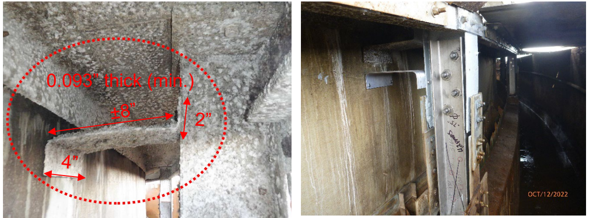
Figure 10: Aluminum angle and "Z" clip providing support to the baffle wall (Typical)
