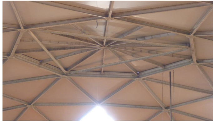
Figure 15: Aluminum stiffeners below the removable dome hatch
