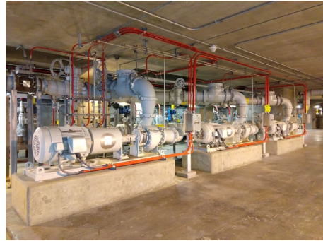
Primary Sludge Pump Replacement
