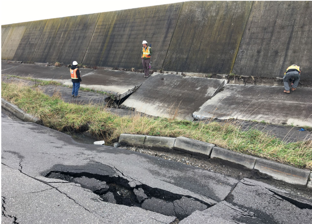
East Tomokomai Port near a coal plant, lateral spread extends 200 ft. inland Hokkaido, Japan, Mag. 6.6, 2018
