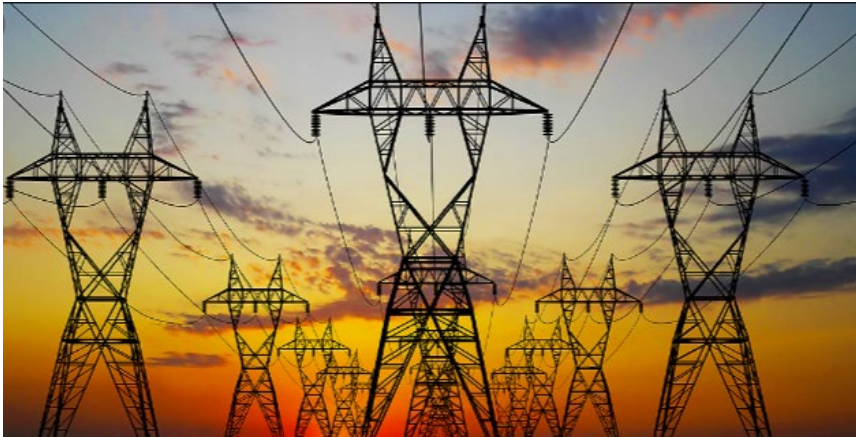
Southern California Edison
