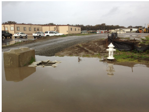
Plant 2 Storm Retention Pond
