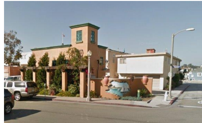
A Street Pump Station
