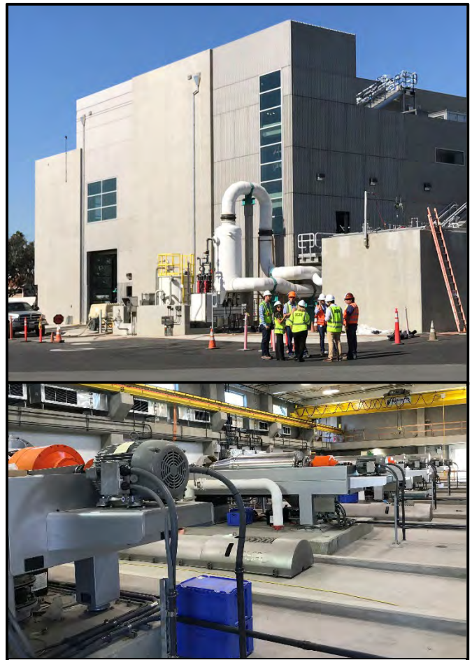
P2-92 Building and Centrifuges
