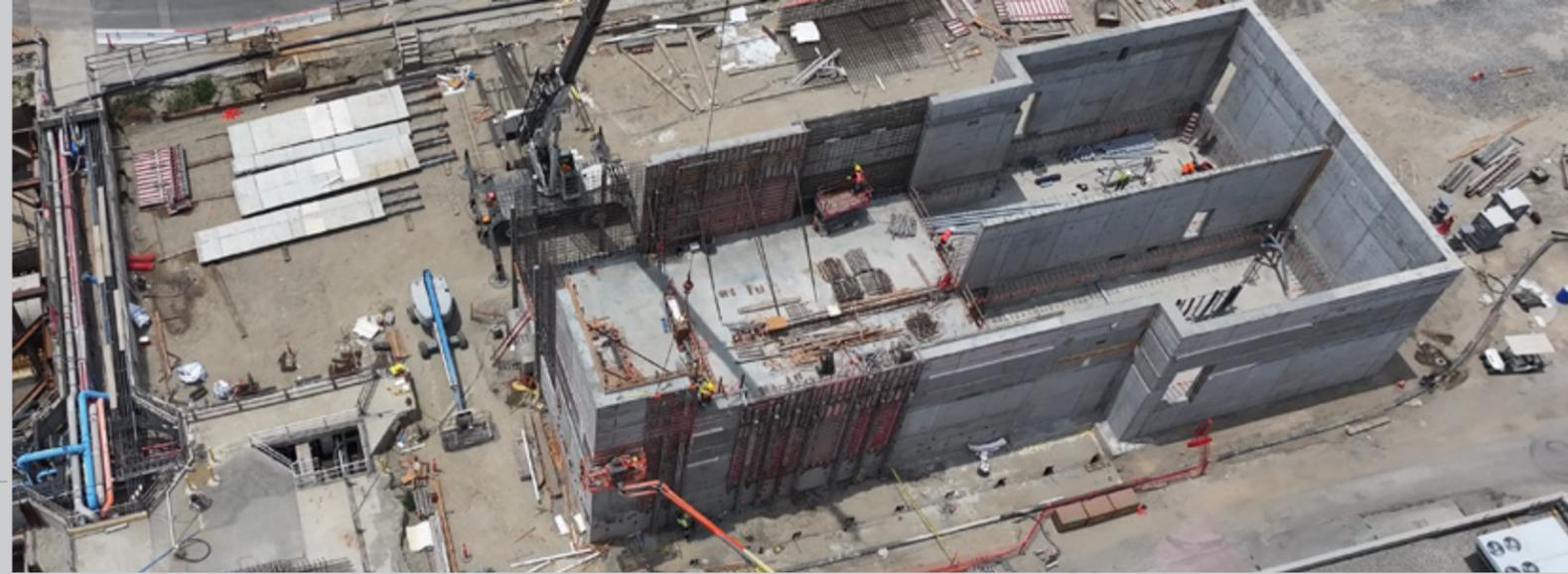
Construction of exterior concrete walls of a new electrical building for the A-Side Primary Clarifiers Replacement, Project No. P2-98A.
