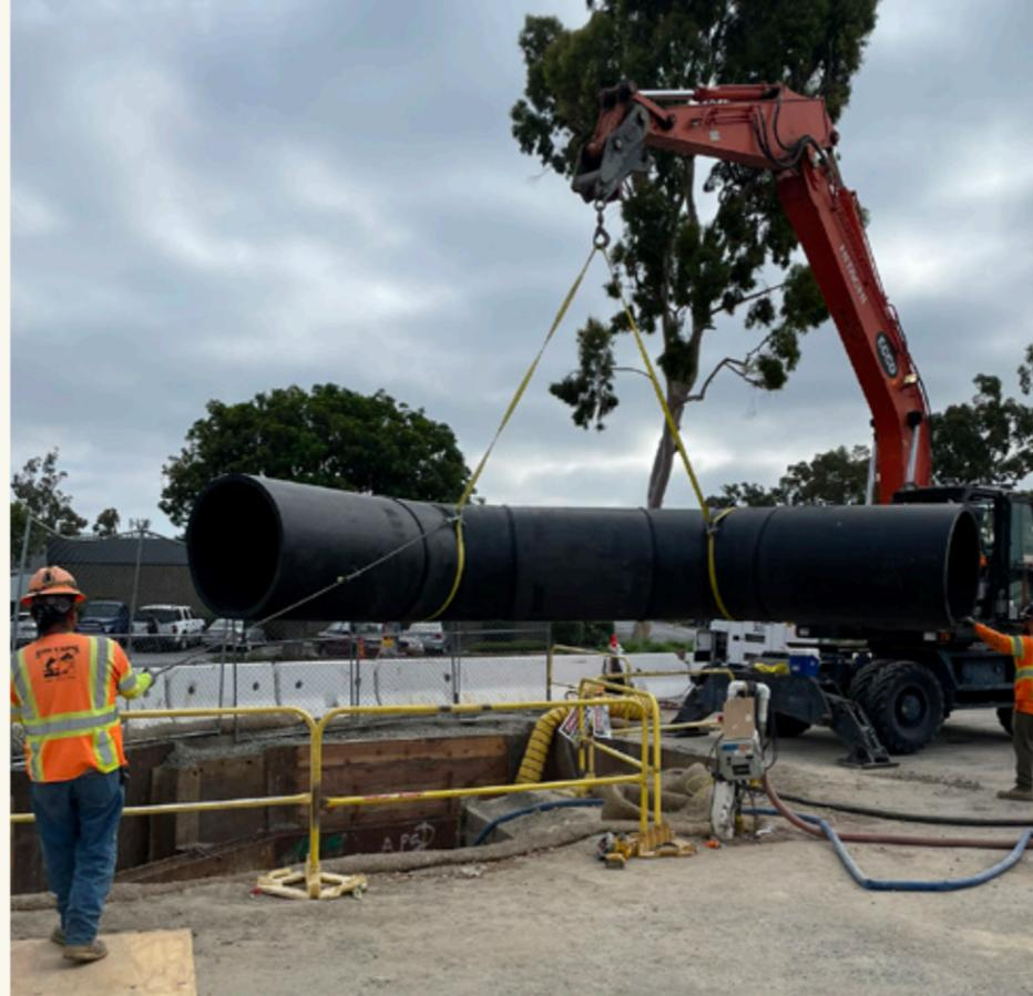
*Installing an angled piece of pipeline on the Baker Force Main Rehabilitation, Project No. 7-65, in the City of Costa Mesa.*
