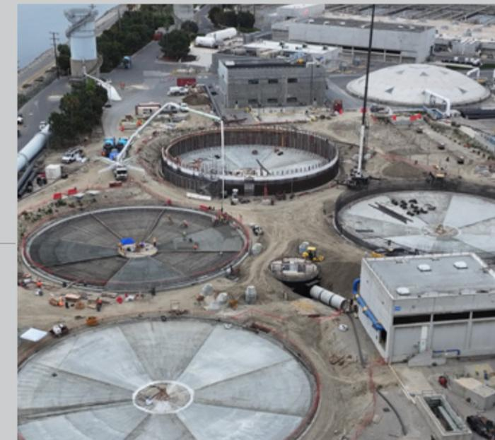
The A-Side Primary Clarifiers Replacement at Plant No. 2, Project No. P2-98A, will construct four new primary clarifiers.
