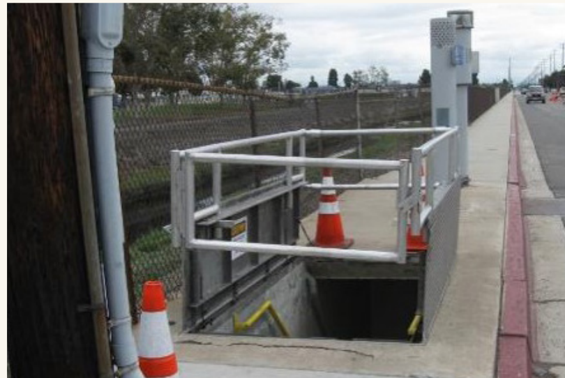
The existing Edinger Pump Station is located completely underground and accessed through a hatch that requires the closure of the sidewalk along a school and park.
