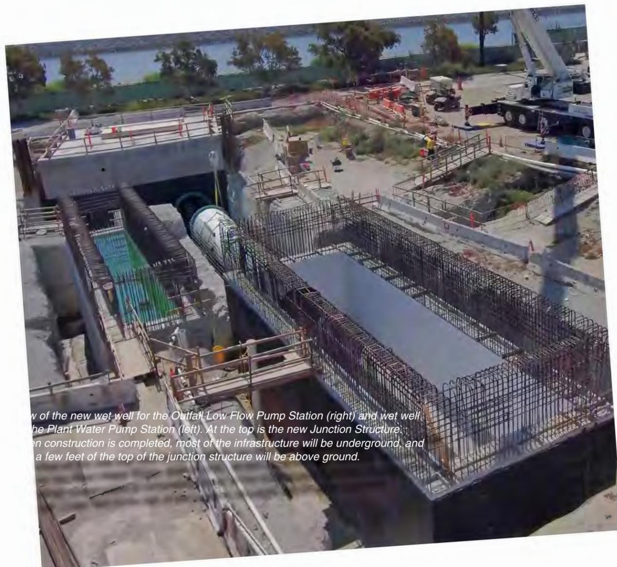
*View of the new wet well for the Outfall Low Flow Pump Station (right) and wet well for the Plant Water Pump Station (left). At the top is the new Junction Structure. When construction is completed, most of the infrastructure will be underground, and a few feet of the top of the junction structure will be above ground.*
