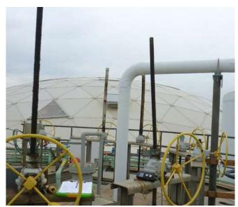
Picture 3: Bent stems and bevel gear operators
