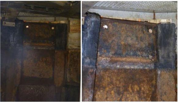
Picture 8: Corroded carbon steel bulkhead from center of distribution structure
