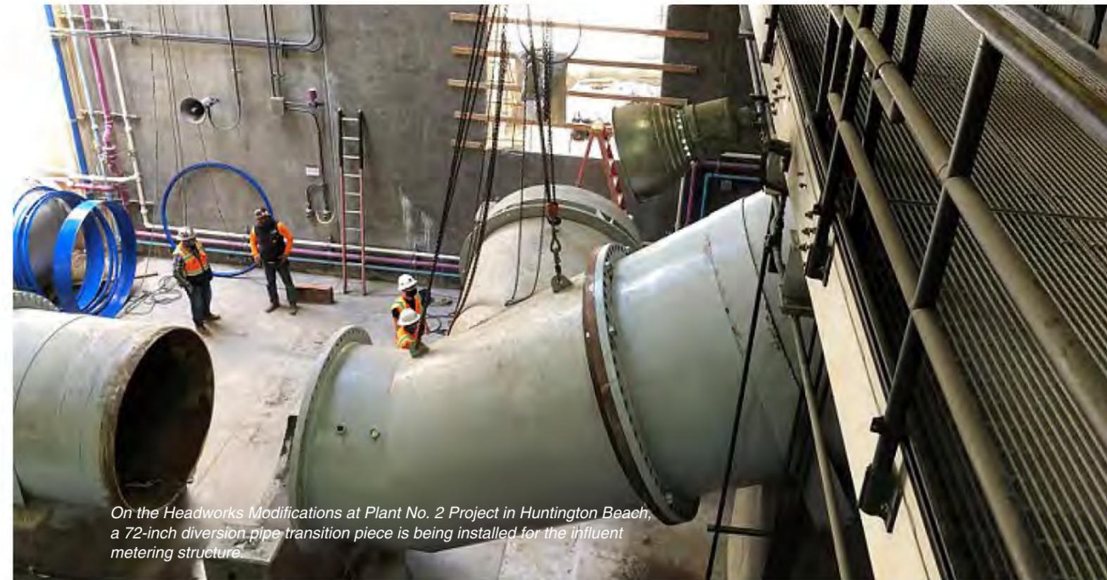
*On the Headworks Modifications at Plant No. 2 Project in Huntington Beach, a 72-inch diversion pipe transition piece is being installed for the influent metering structure.*
