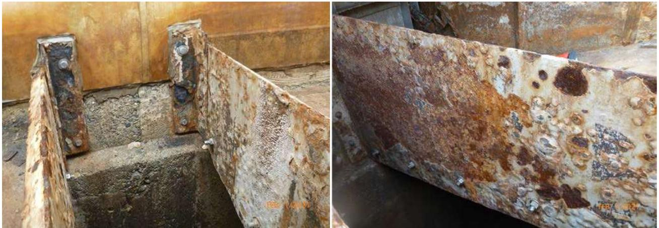
Picture 12: Corroded steel weir plates
