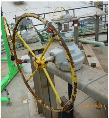
Picture 4: Corroded handwheel and bevel gear operator
