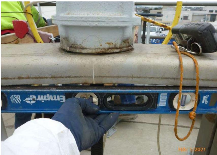
Picture 5: Bent gate top frame
