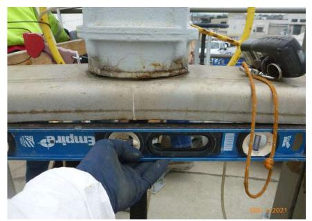
Picture 5: Bent gate top frame
