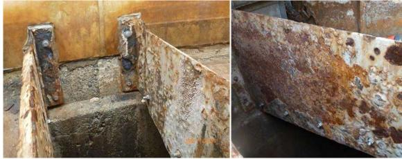
Picture 12: Corroded steel weir plates
