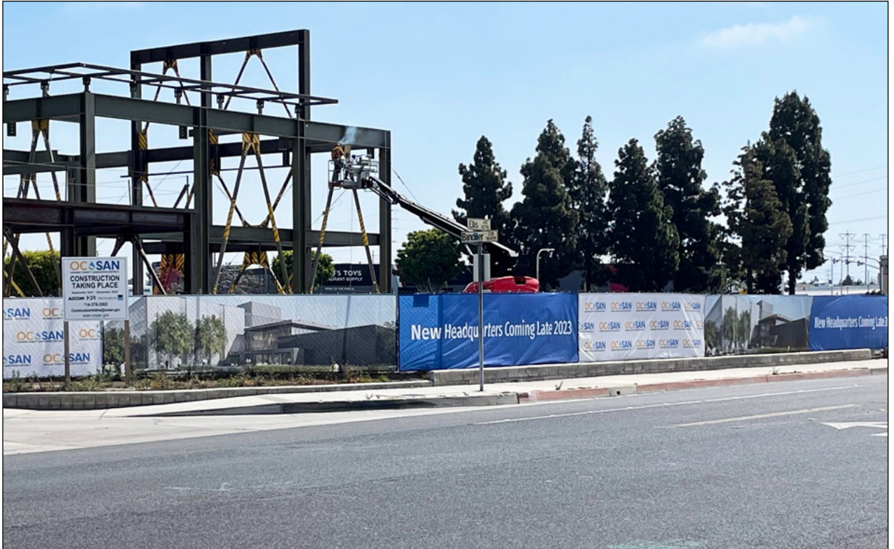
Headquarters Construction Fence Graphics
