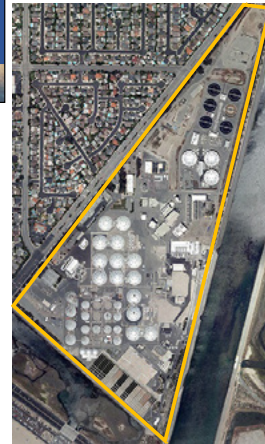
Treatment Plant No. 2 Huntington Beach
