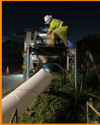
Gravity Rehabilitation Using Cured-in-Place-Pipe
