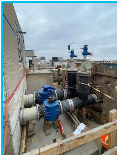
Valve Vault Replacement
