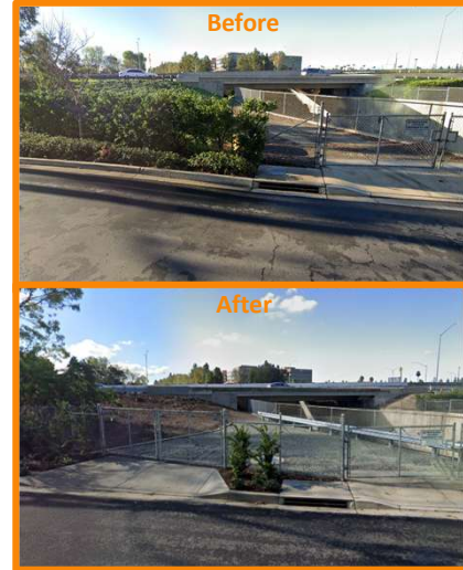
Manhole Access Improvements
