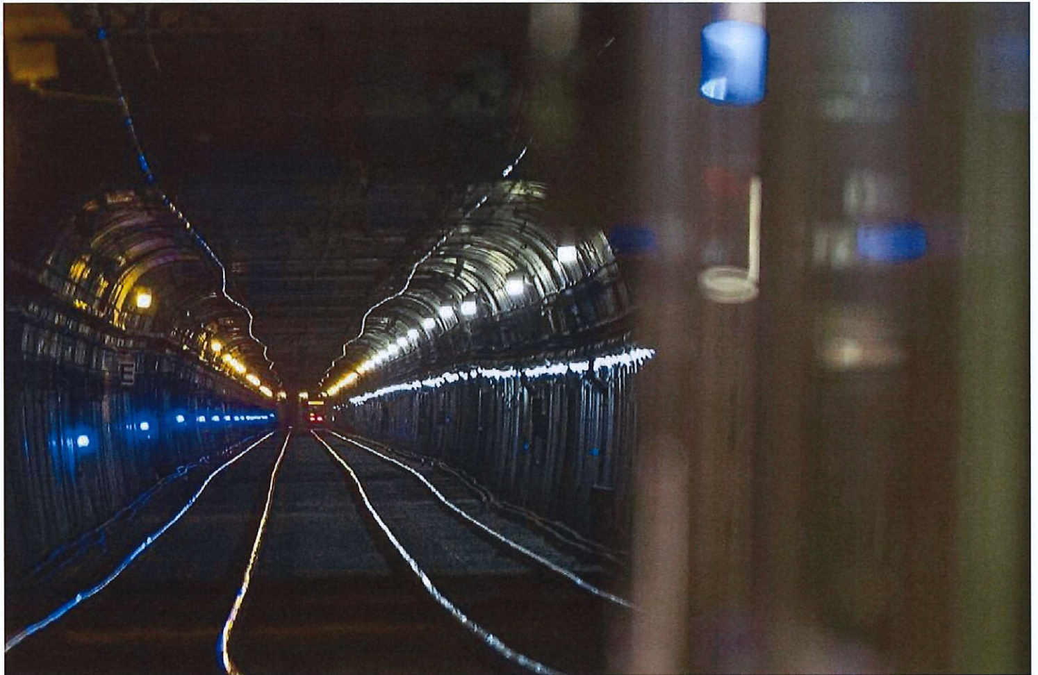
The Twin Peaks Tunnel
