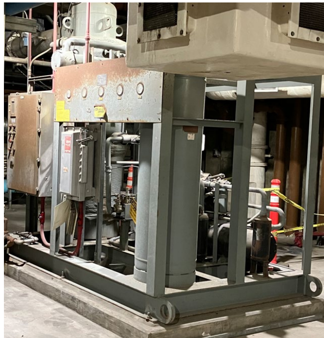
Figure 1: Refrigerated gas dryer skid located in the basement of Plant No. 1 Gas Compressor Building. The unit is currently inoperable.
