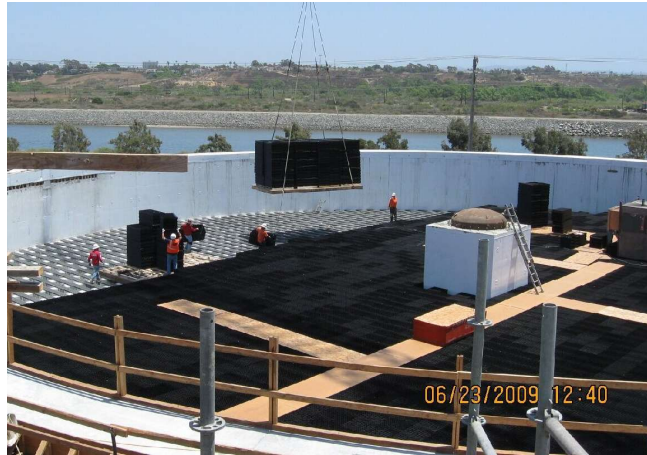
Media Installation at Plant No. 2
