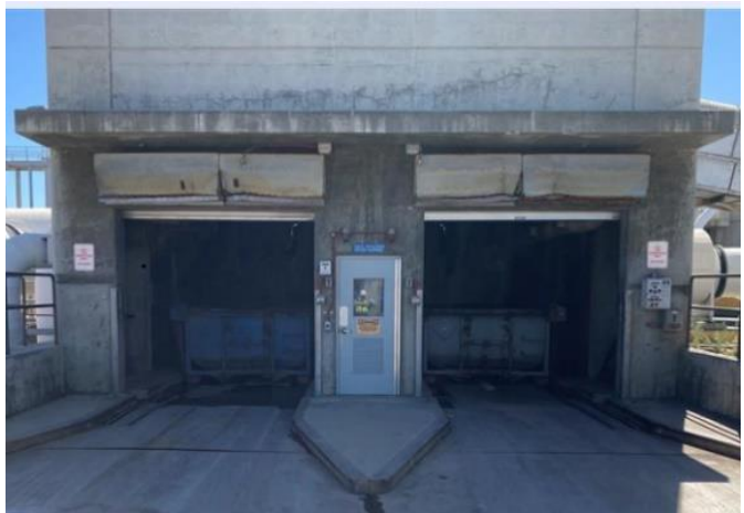
Photo of Plant No. 1 Grit and Screening Area
