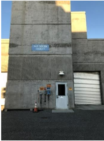
Photo of Plant No. 2 Screening Area
