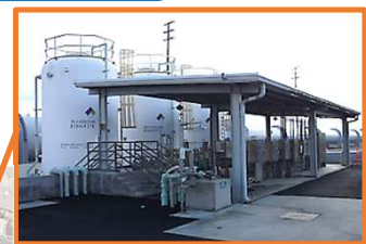
Sodium Bisulfite Station Dechlorination for long outfall (when needed) and short outfall (when in use)
