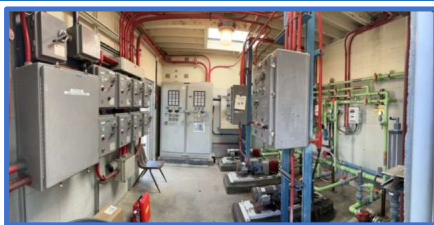
Anionic Polymer Station Used for primary treatment to settle solids
