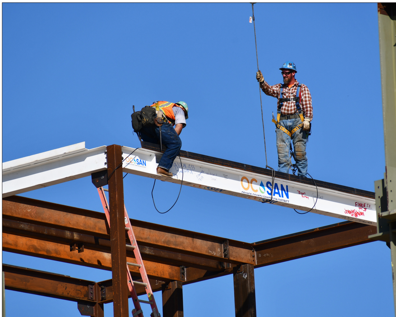
Final steel beam installation at Headquarter Complex.
