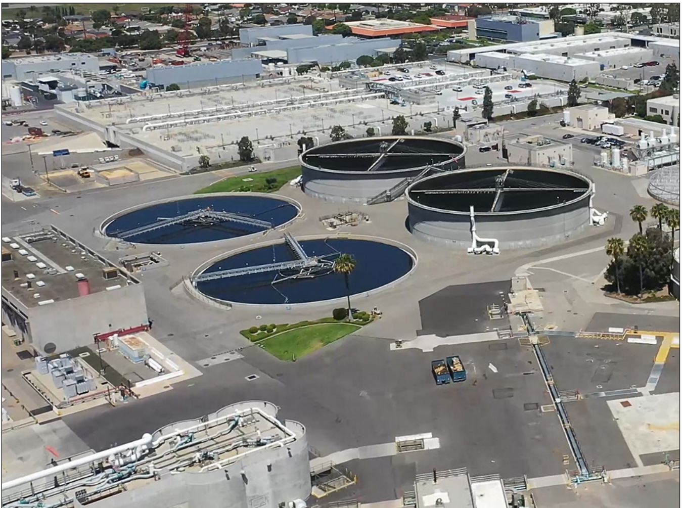
Reclamation Plant No. 1 in Fountain Valley.
