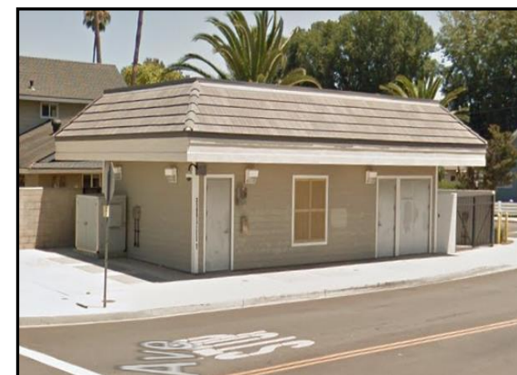
College Pump Station
