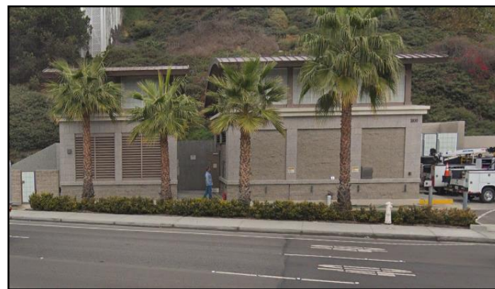
Rocky Point Pump Station
