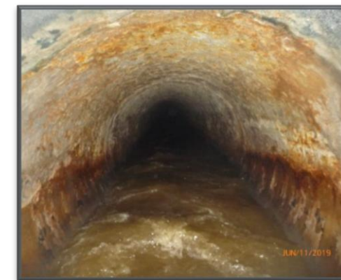
Santa Ana Trunk Sewer
