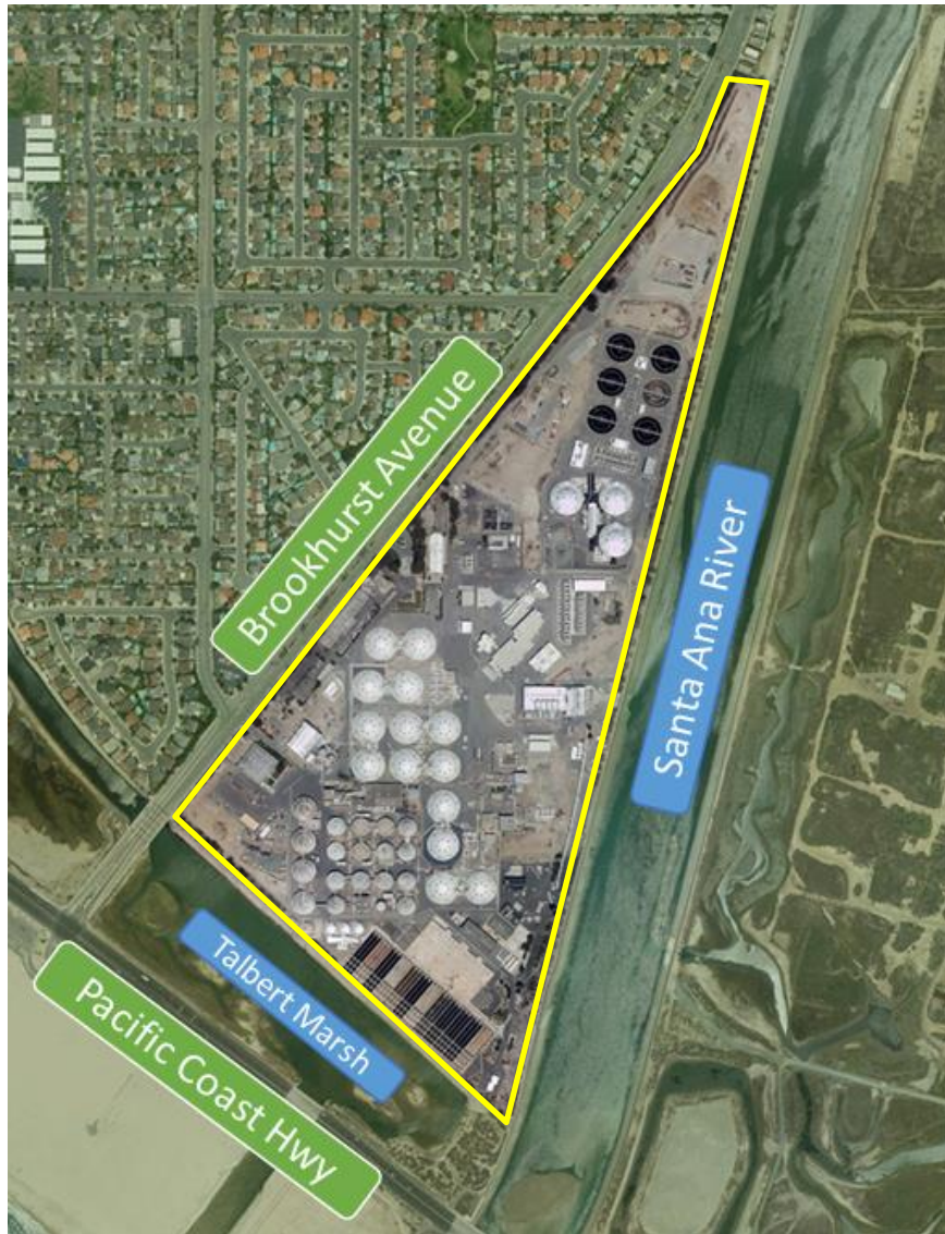
Figure 2.3. Aerial View of Treatment Plant No. 2
