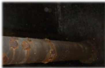
Corroded Piping
