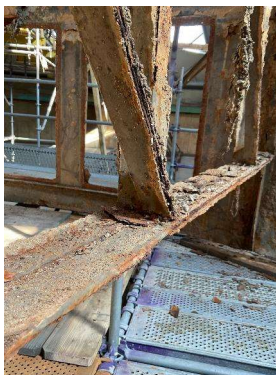
Condition of steel before sandblasting
