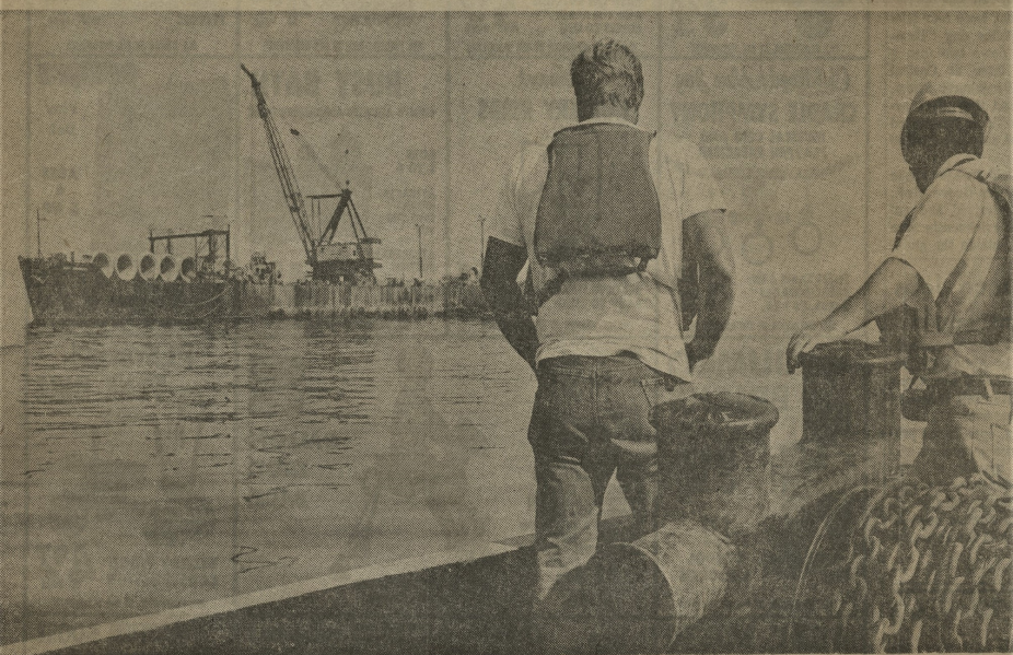
65-TON PIPE SECTIONS LINE DECK OF WORKSHIP DAVEY CROCKET
