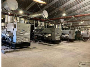
Multiple 2,000kW Standby Generators
