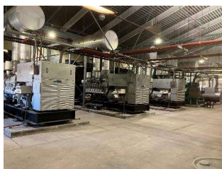
Multiple 2,000kW Standby Generators
