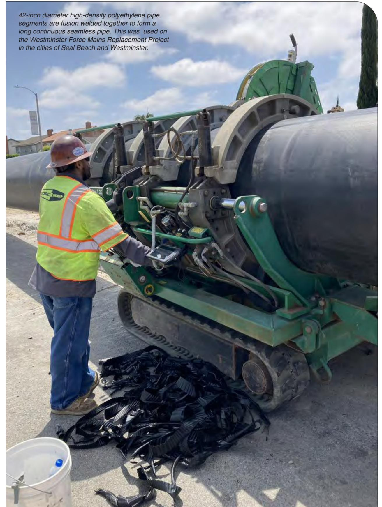
42-inch diameter high-density polyethylene pipe segments are fusion welded together to form a long continuous seamless pipe. This was used on the Westminster Force Mains Replacement Project in the cities of Seal Beach and Westminster.
