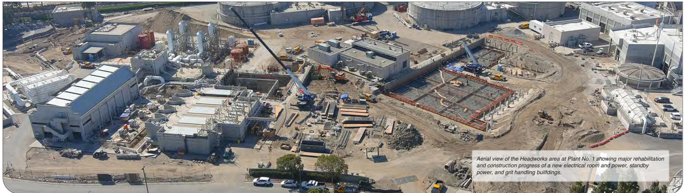
Aerial view of the Headworks area at Plant No. 1 showing major rehabilitation and construction progress of a new electrical room and power, standby power, and grit handling buildings.
