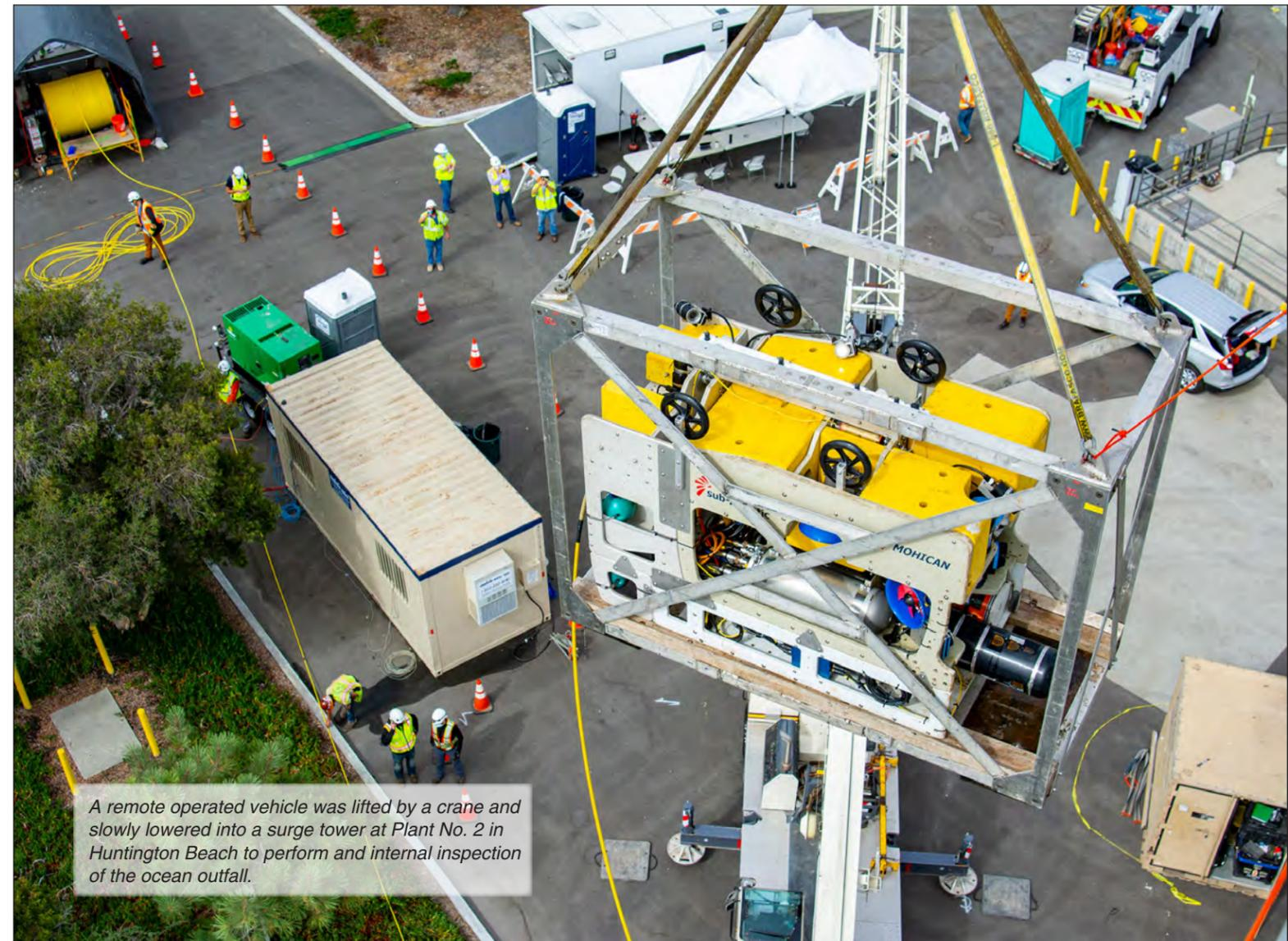
*A remote operated vehicle was lifted by a crane and slowly lowered into a surge tower at Plant No. 2 in Huntington Beach to perform an internal inspection of the ocean outfall.*
