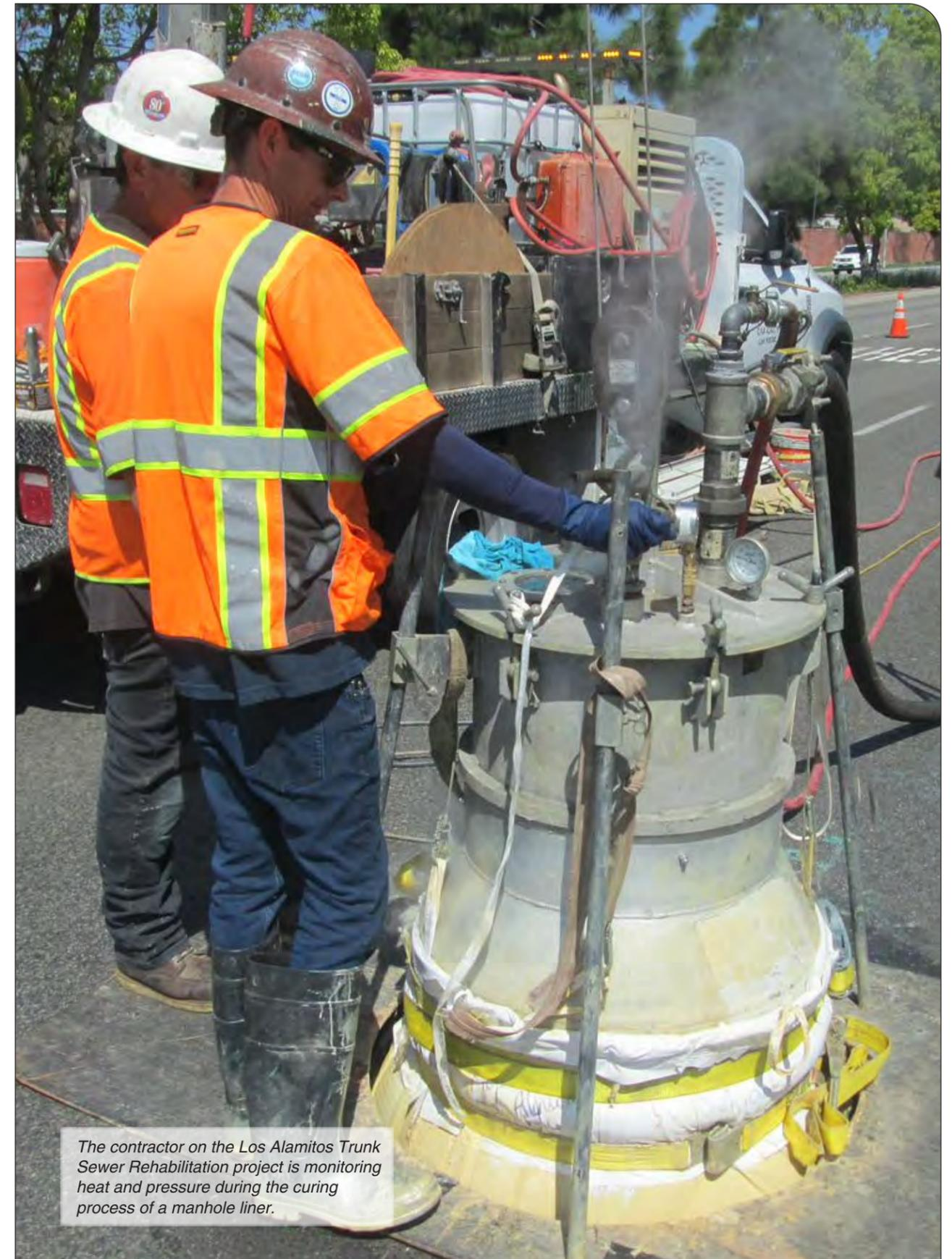
*The contractor on the Los Alamitos Trunk Sewer Rehabilitation project is monitoring heat and pressure during the curing process of a manhole liner.*
