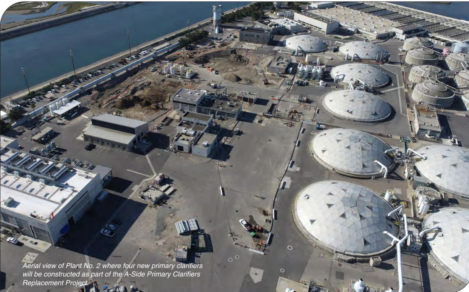
*Aerial view of Plant No. 2 where four new primary clarifiers will be constructed as part of the A-Side Primary Clarifiers Replacement Project.*
