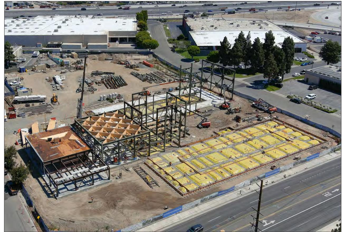
*The foundation work is completed and vertical structural steel elements and mass timber are starting to go up on the Headquarters Complex Project.*
