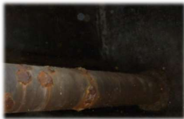
Corroded Piping
