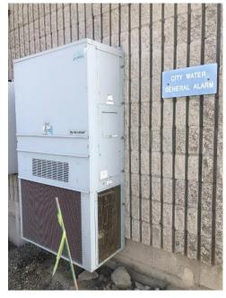
Figure 3: The P2 Gas Compressor roof top unit is corroded and are at the end of their service life.
