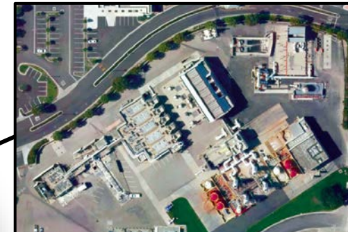
P1-105 Headworks Rehabilitation and Expansion at Plant No. 1 Project Budget: $406M Bid Opening: 12/15/20
