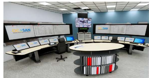
J-120A Control Room Reconfiguration
