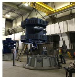
Effective Project Execution
