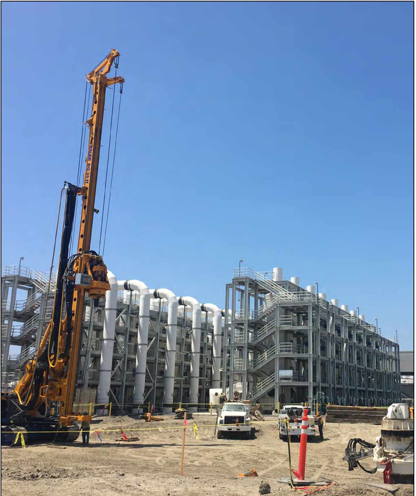
Deep Soil Mixing Rig at Plant No. 2 in Huntington Beach
