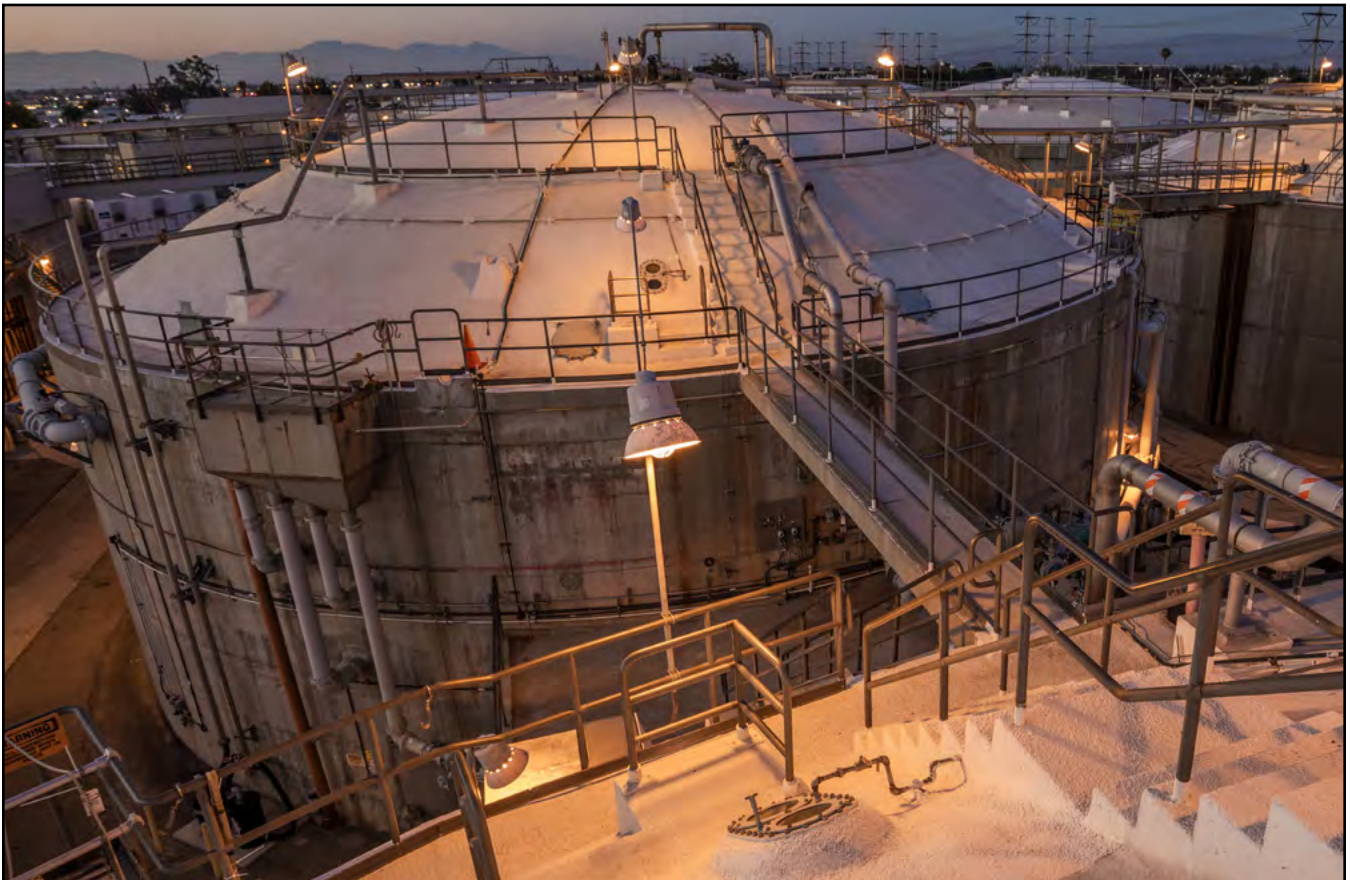
Digesters at Plant No. 1 in Fountain Valley
