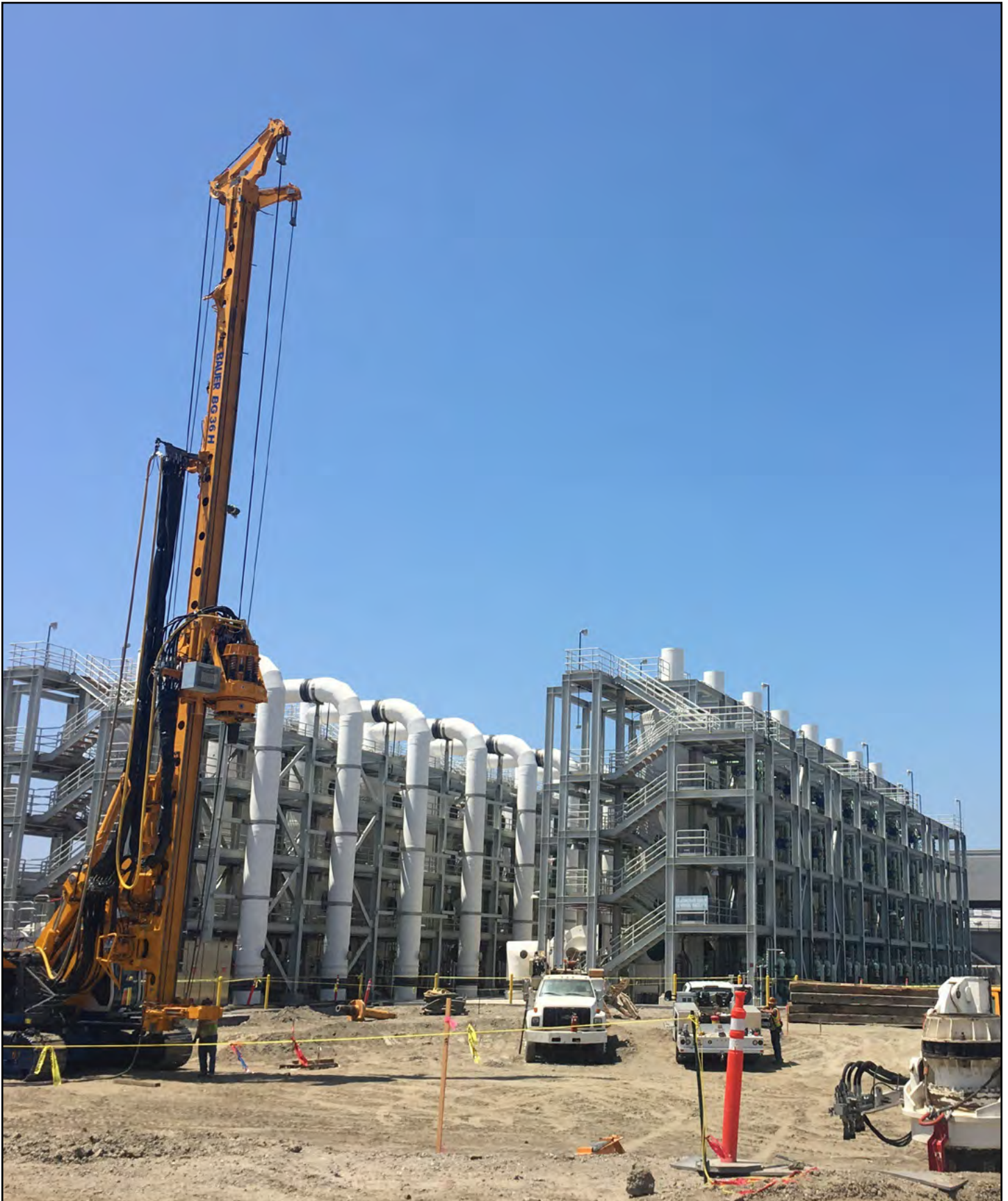
Deep Soil Mixing Rig at Plant No. 2 in Huntington Beach
