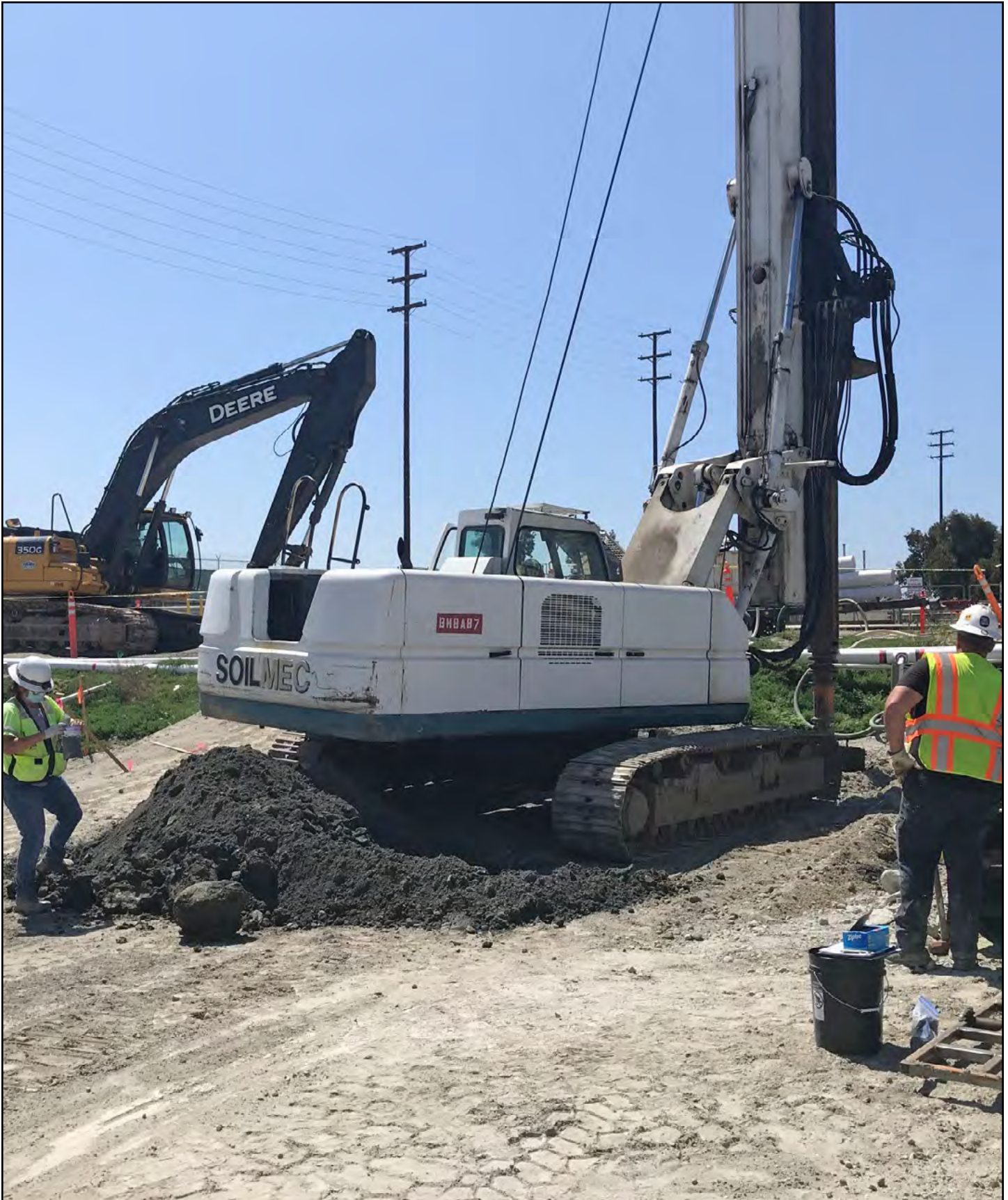
Redrilling well at Plant No.2 in Huntington Beach
