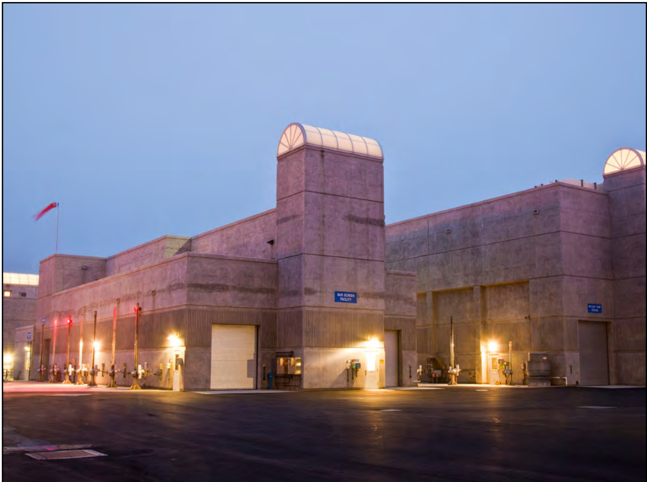
Bar Screen Facility and Influent Pump Station at Plant No. 2 in Huntington Beach
