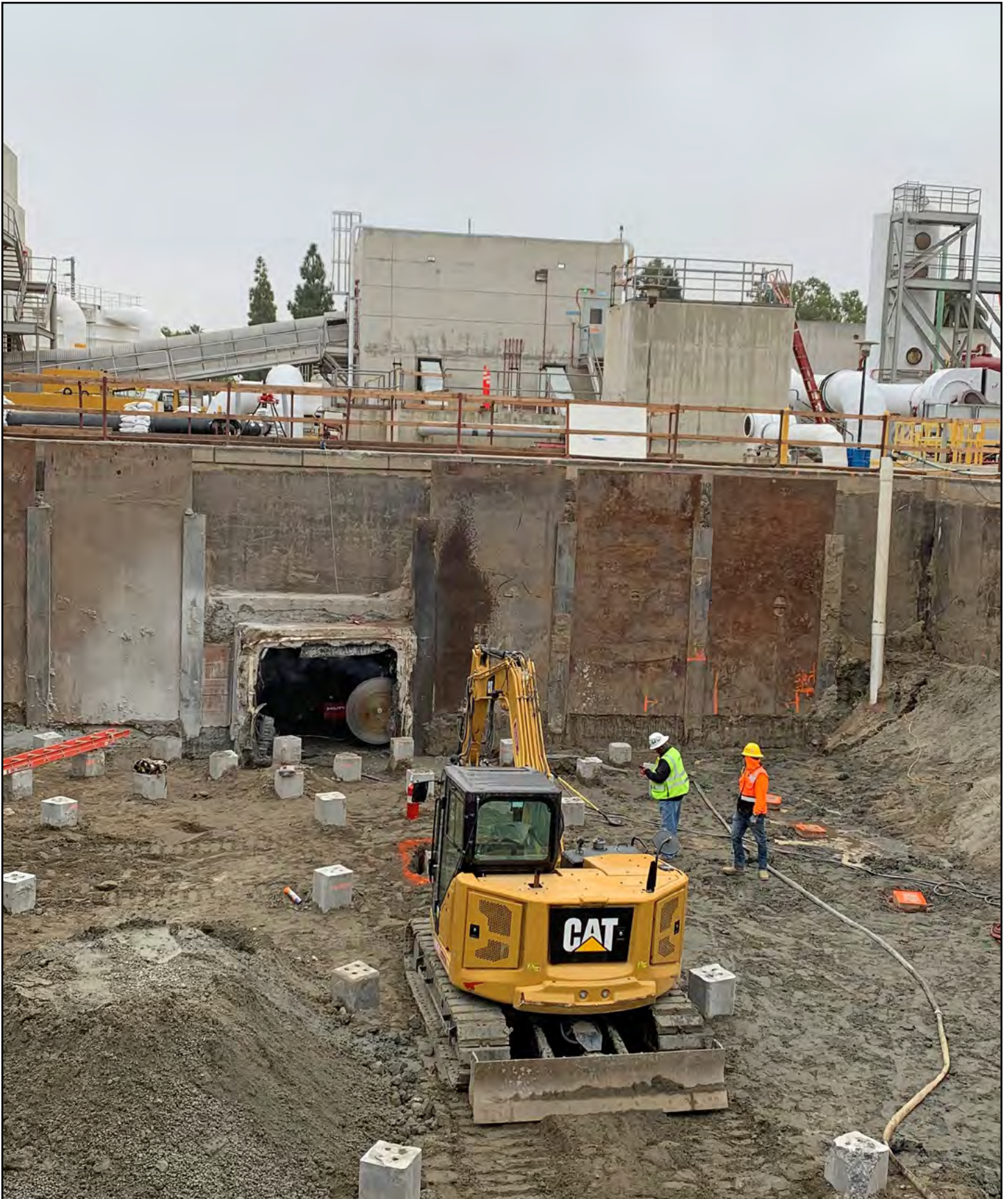
Headworks Rehab Construction at Plant No. 1 in Fountain Valley
