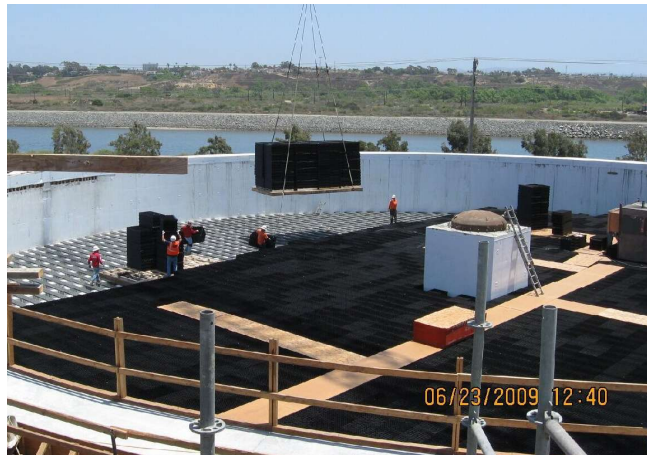
Media Installation at Plant No. 2
