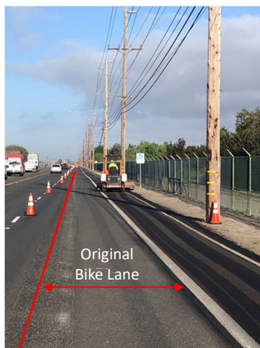
Temporary Bike Lane
